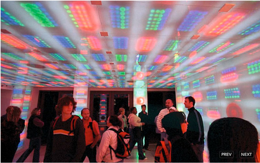
Fig. 5 The Breezeway at Rockefeller Center by Electroland, in which LED lighting is controlled based on the movement of visitors, as sensed by a 3D camera-based personnel-tracking system. (photo by Electroland)
