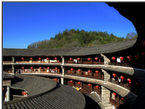
Fig. 1. Fujian Hakka Earth architecture
