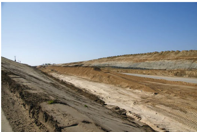
Fig. 5 The view of direct channel construction
