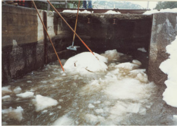
Fig. 9 Guiding an ice bolus out of the exit of an inverted siphon
