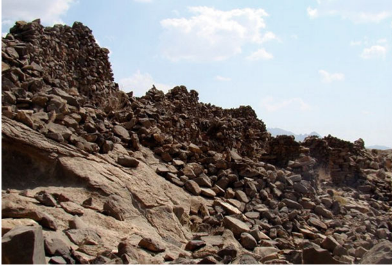
Fig. 6.38 Typical Iron Age hill top fortress with surrounding dry stone walls (photo by Jill Newby)
