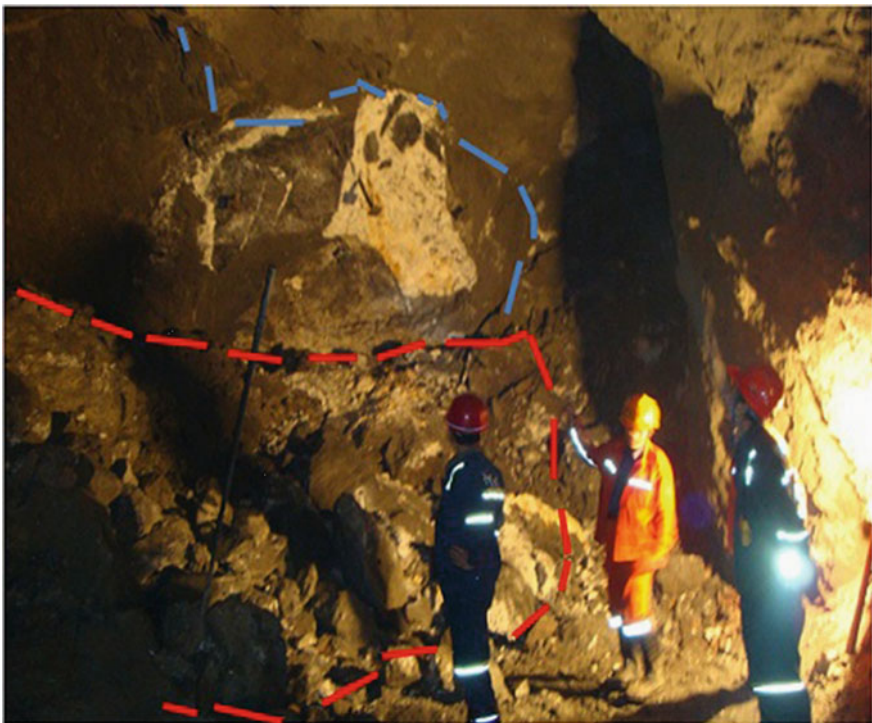
Fig. 9.7 Collapse in 2# tunnel. With kind permission from “PERGAMON-ELSEVIER SCIENCE LTD”: Fig. 5, Wang (2014). All rights reserved
