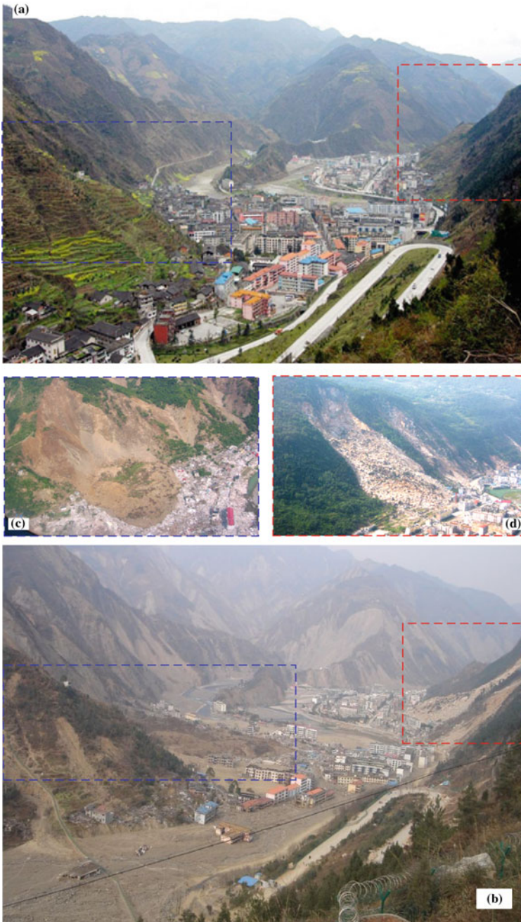
Fig. 1.2 Comparison of Beichuan County before (a) and after (b) the Wenchuan earthquake. The earthquake induced two catastrophic landslides, c new Beichuan middle school landslide, it destroyed the school and killed 907 people, most of them were students, and d Wangjiayan landslide, it buried the old town and killed at least 1600 people (Photographs are from Tang) identify the landslide prone slopes as well as their affected areas first
