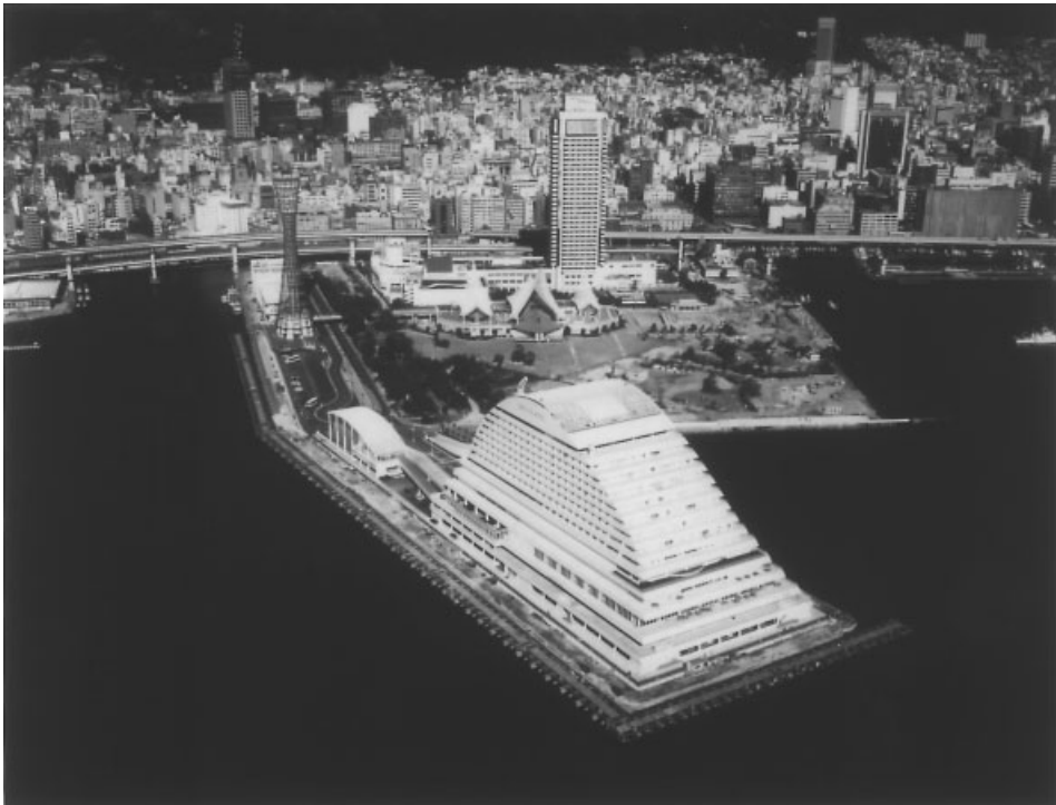
Fig. 5.7 This wharf at Nakatotsu in Japan was heavily damaged during the Kobe Great Earthquake in 1995. The rehabilitation project involved dredging, piling and the development of this futuristic building. (Photo courtesy of Penta Ocean Construction, Tokyo, Japan)
