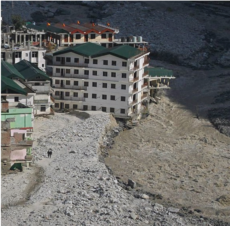
Fig. 5.4 Construction of buildings on riverbed in Joshimath, Uttarakhand, violating infrastructure norms (Picture taken by author post Uttarakhand Disaster in 2013)
