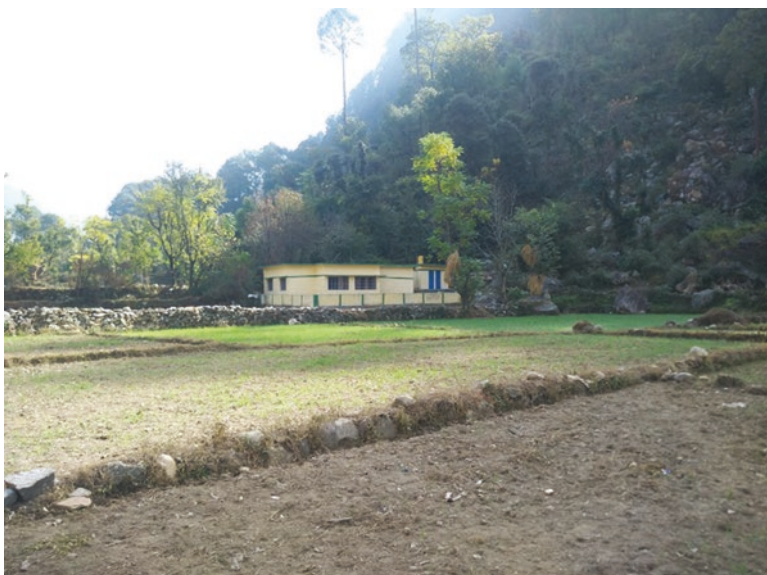
Fig. 15.1 A reconstructed school in Uttarkashi, which was washed away during a flash flood in 2013
