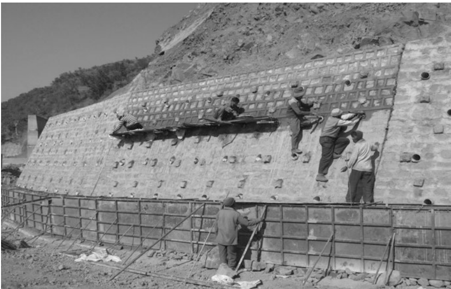
Fig. 19.1 Rubble masonry gravity retaining wall along national highway, Himachal Pradesh, India
