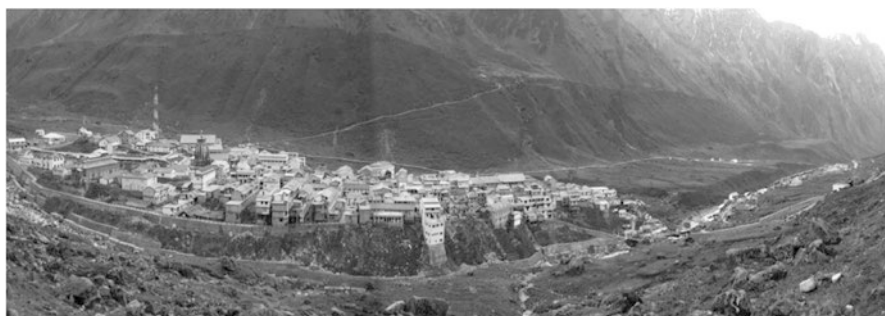
Fig. 9.2 View of the temple township of Kedarnath, with camera looking east
