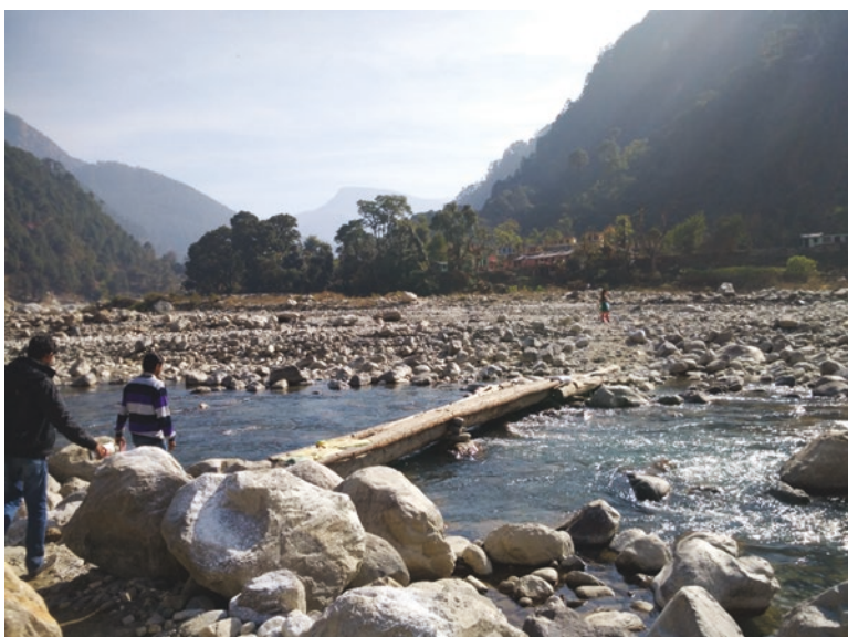
Fig. 15.2 The main approach road to a school in Uttarkashi
