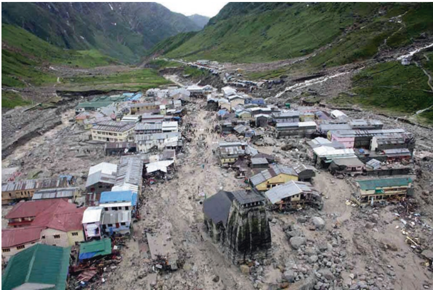
Fig. 5.1 Construction of infrastructure just below the fragile glacial lake Chorabari Tal, Kedarnath (Indian Army Aviation July 2013 post-disaster photograph)
