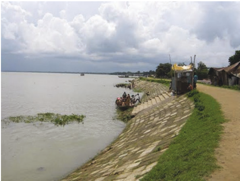
Fig. 8.3 Strengthening of embankments in flood-prone areas
