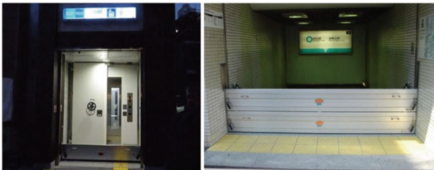
Fig. 8.16 Water tight doors at the entrance of the subway (By courtesy of Tokyo Metro Co., Ltd.)
