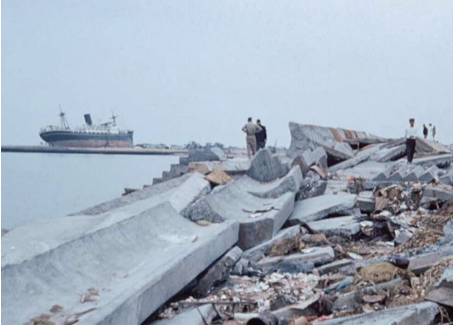
Fig. 8.11 Concrete seawall hit by the storm surge caused by Isewan Typhoon (Typhoon Vera) in 1959 and a wrecked large ship after uncontrollable drift (By courtesy of Professor Yoshiaki Kawata, Photo taken by the late Professor Yuichi Iwagaki)
