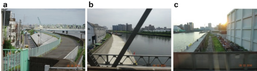
Fig. 8.15 (a-c) Ground surface lower than the water level of the river
