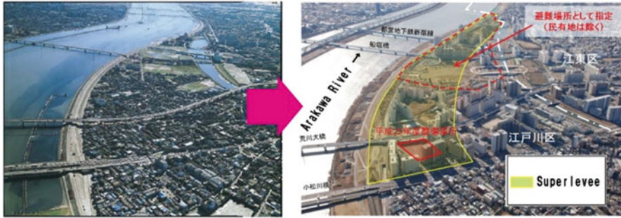
Fig. 8.23 Super levee before and after placement (By courtesy of Kanto Regional Development Bureau)
