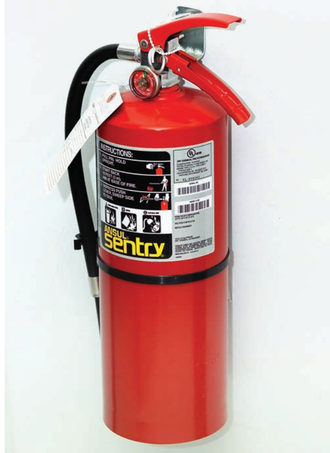
FIGURE 5-8 Typical fire extinguisher with tag indicating when last serviced.
