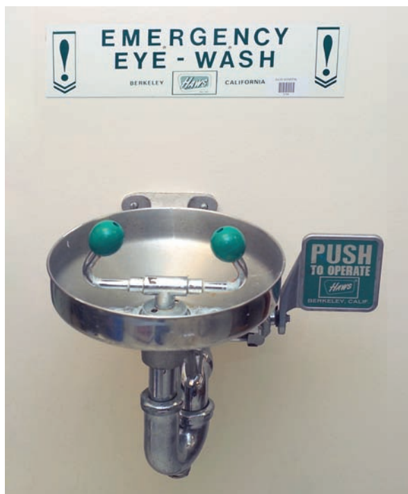
FIGURE 5-11 Eyewash station for emergency incidents involving biohazards and toxic chemicals. Source: Delmar/Cengage Learning.
