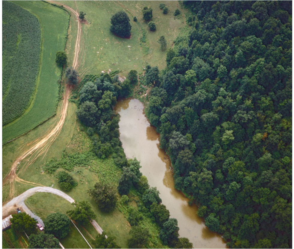
Fig. 3.28 Aerial photo showing the head spring of Indian Creek south of Union
