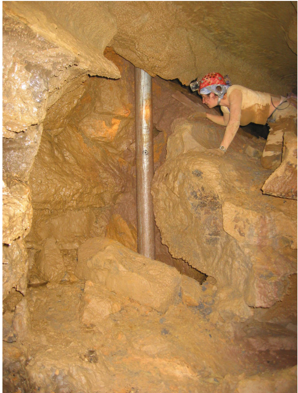
Fig. 16.8 Steel well casing from domestic well intersecting passage in Scoop City section of the cave. Photo by I.D. Sasowsky
