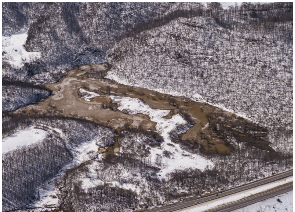
Fig. 12.9 Aerial photograph showing Interstate Lake ponded to a depth of 50 ft on March 8, 2015. Photograph by W.K. Jones
