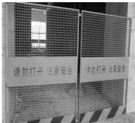
Figure 10. Elevator entrance limb protection.
