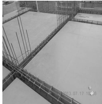
Figure 2. Beams and slab formwork installation.
