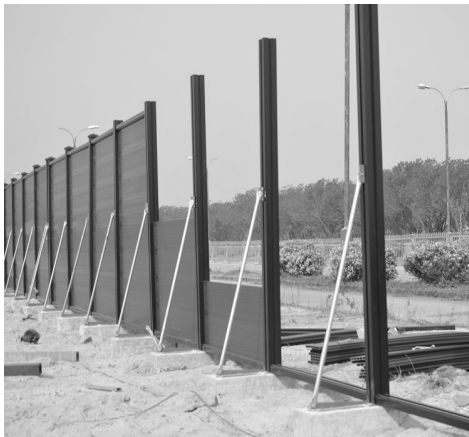
Figure 6. Recycled fence assembling.
