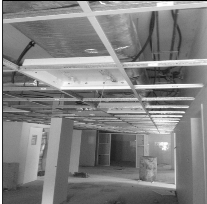
Figure 6. Medical gazes installation in ceilings.
