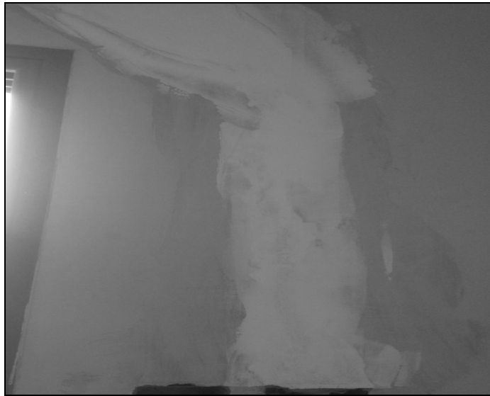
Figure 3. Preparing walls for maintenance.
