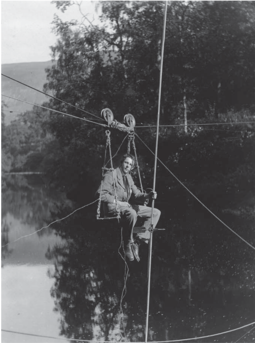
River current meter gauging from a 'bosun's chair' – Invergarry 1913: Some of the earliest river gauging in the UK was carried out by Captain William Newsam McClean in 1913, when he installed a water level gauge on the River Garry, close to the lodge of Invergarry House, Inverness-shire. He subsequently set up gauging stations and raingauges across the River Ness basin. With a strong desire to see large-scale hydro power established in the Scottish Highlands as a means of stimulating economic and social development, McClean used his own resources to establish a hydrological survey that was truly ahead of its time. The appointment of an Inland Water Survey Committee in 1935 was likely, in no small part, to have been due to his efforts. (Source: Reproduced with permission of Dundee University.)
