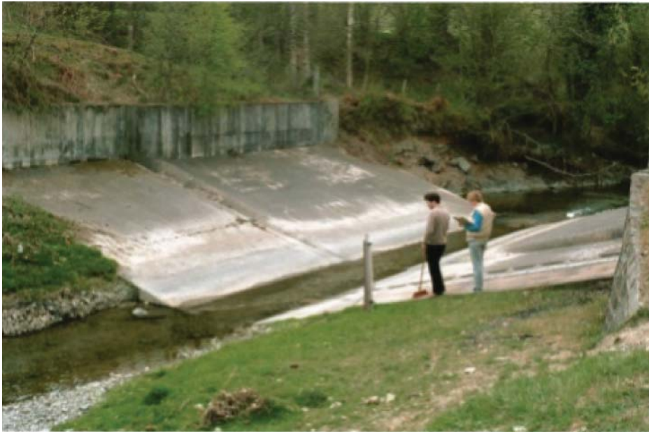
Fig. 11.9 Large capacity flume at Rhos-y-Pentref in central Wales (Photo: NRFA.) (Source: Reproduced with permission of CEH.)
