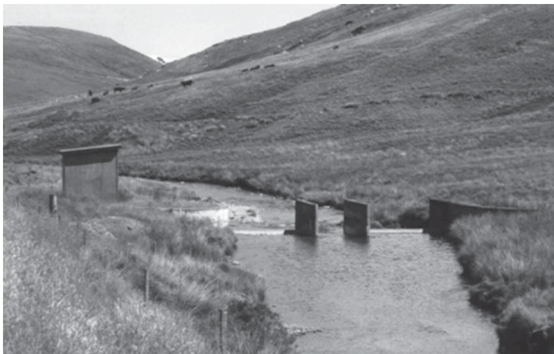
Fig. 2.16 Compound Crump weir in the Wye. (Source: Reproduced with permission of CEH.)
