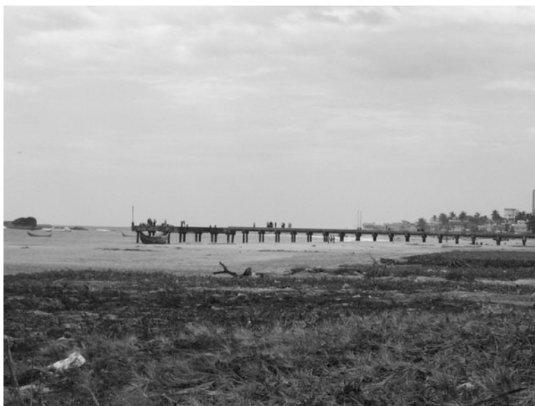
Photo 5.4 Undamaged jetty at Colachel
