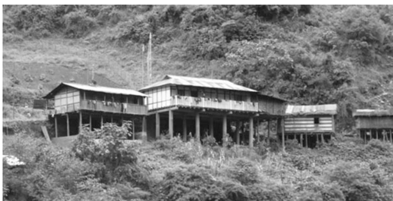
Fig. 14.4 A typical timber construction in the hills of North India- Ground storey for cattle and upper storey for self
