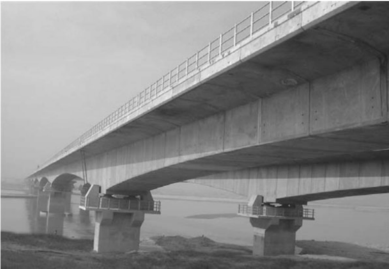
Fig. 10.11 Allahabad bypass bridge over river Ganga, Allahabad
