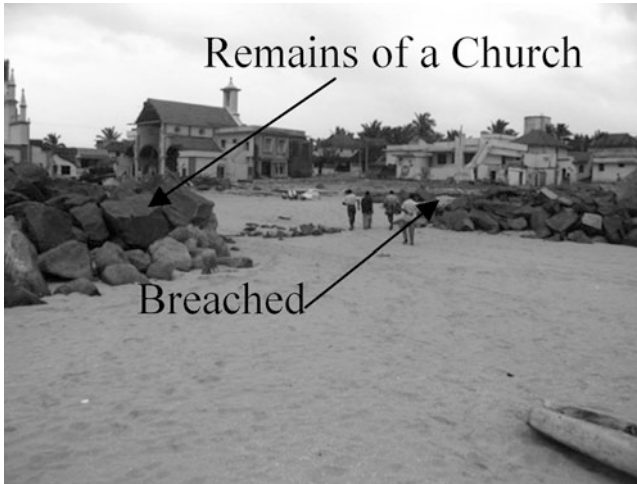
Photo 5.2 Damaged Seawall and Church at Kezhaamanakudithurai
