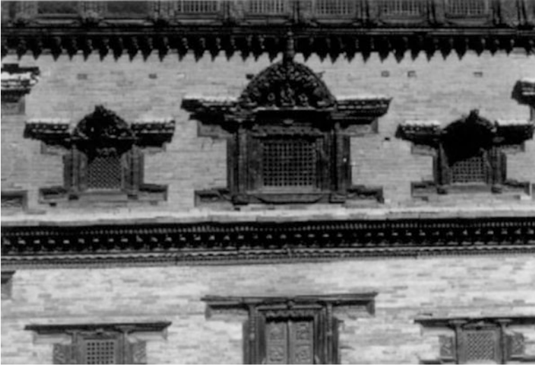
Fig. 14.1 Timber bands in Kathmandu Palace
