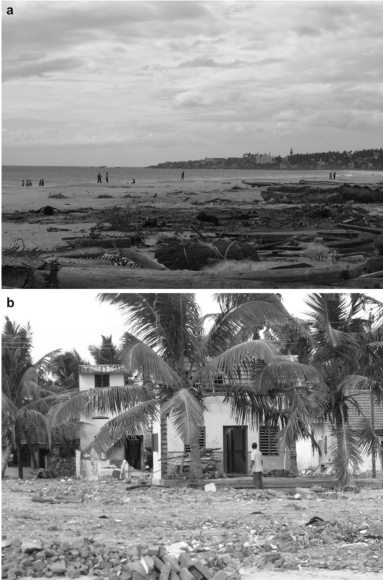
Photo 5.5 (a, b) Damage to residential buildings at Pillathopputhurai
