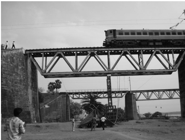
Fig. 15.1 Photograph of bridge
