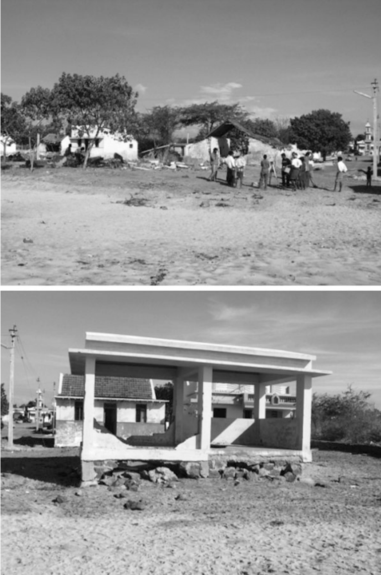
Photo 5.6 Damaged residential buildings at Kootapuli
