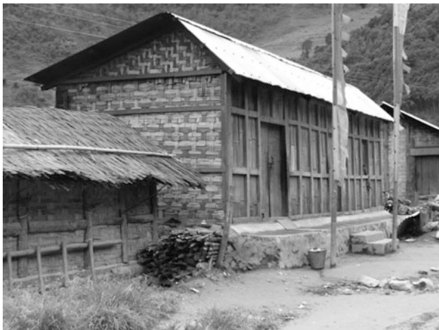
Fig. 14.3 A typical timber hut with walls made of bamboo mats in North East India
