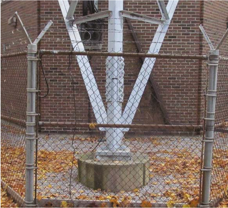
Fig. 2. One of the caisson foundations to be retrofitted
