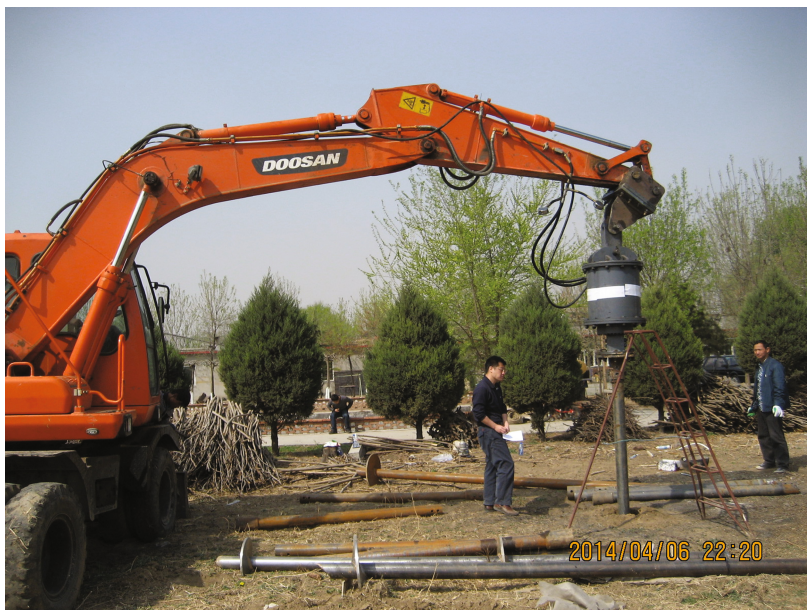
Fig. 1. Installation of screw piles
