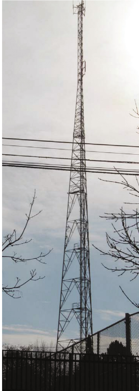
Fig. 1. The self-supporting tower examined
