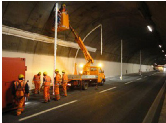
Fig. 3.15 Activity of positioning underprops through the use of a hydraulic basket
