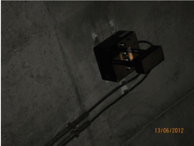
Fig. 3.11 Picture of one of the anemometers belonging to the tunnel ordinary equipment
