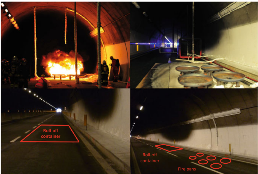
Fig. 4.2 Effect of obstacle on the smoke dispersion after the two fire tests
