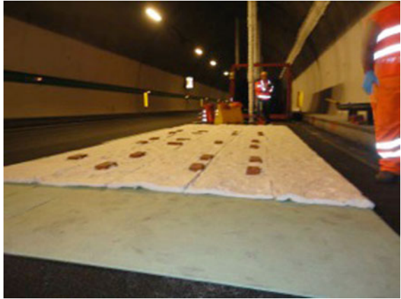
Fig. 3.19 Second insulation layer of alkaline earth silicate wool
