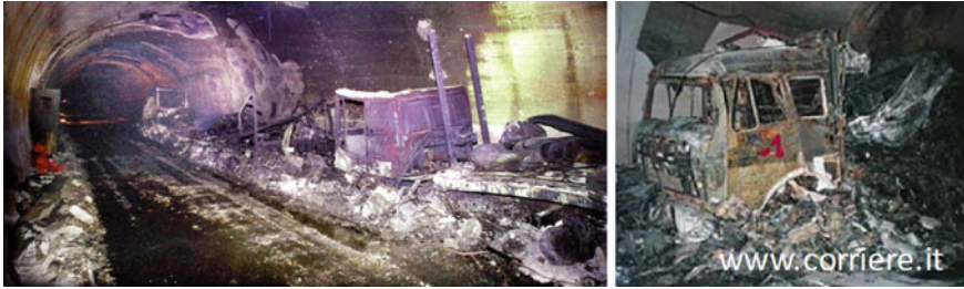
Fig. 1.1 Pictures of the accident occurred in the Mont Blanc Tunnel (1999)
