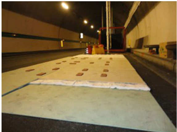
Fig. 3.20 Third insulation layer with gypsum plasterboards
