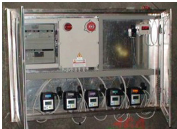
Fig. 3.10 Box containing the instruments used for real-time monitoring of the air quality in the observers area
