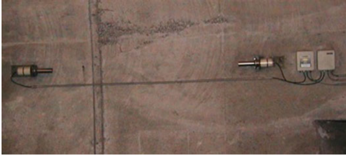
Fig. 3.24 Smoke opacimeter and CO detector located on the tunnel wall (model CODEL TunnelCraft AQM CO+VIS)
