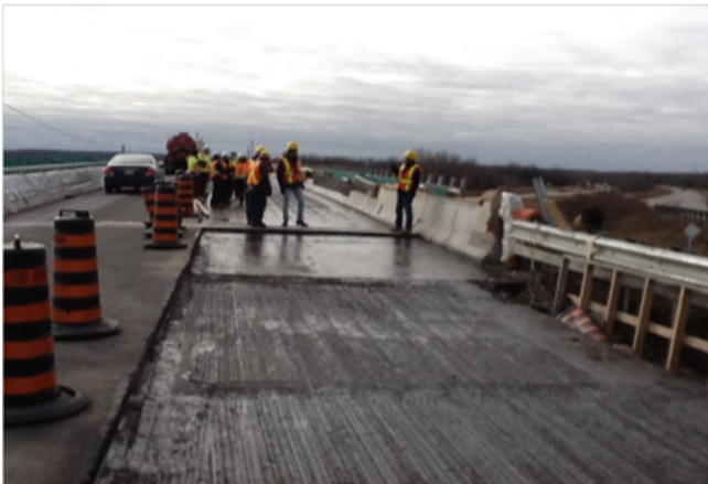
Fig. 3. The Highway 34 Bridge
