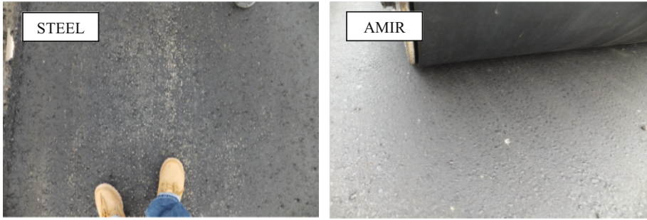
Fig. 12. Finished asphalt deck surface, Highway 34 Bridge
