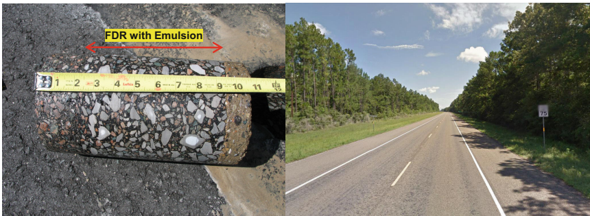
Fig. 2. Successful FDR project that maintain low IRI for the last 10 years
