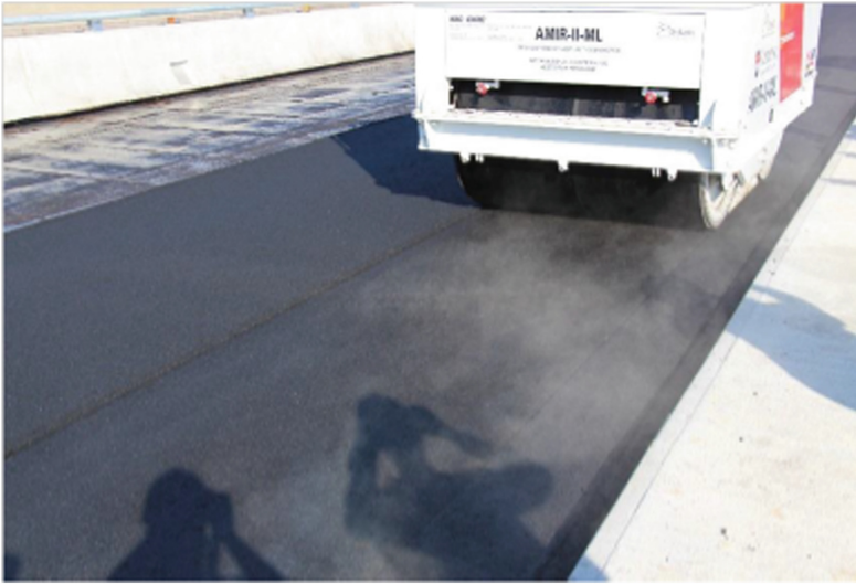
Fig. 7. AMIR compacts the first lane, Holt Road Bridge
