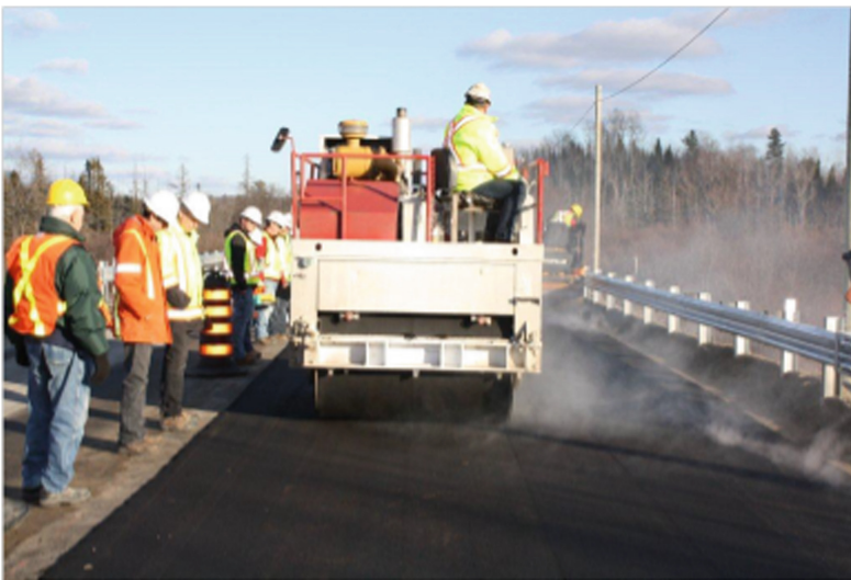
Fig. 8. AMIR compacts its lane of the Distress River Bridge
