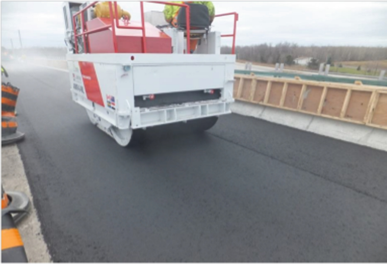
Fig. 4. AMIR-II compacts Highway 34 Bridge deck
