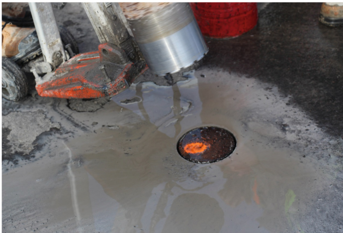
Fig. 10. Extraction of cores
