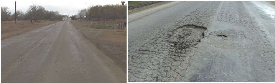
Fig. 5. Existing pavement conditions on US99 before FDR
