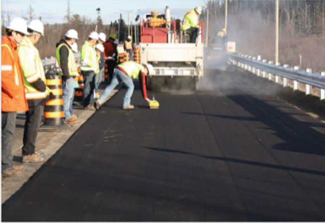
Fig. 11. Measuring of relative compaction behind AMIR
