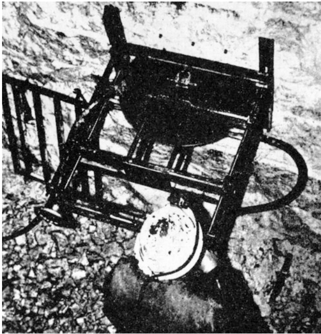
Fig. 15 In situ stress measurement using flat-jack in the 1970s in France (after Hoek 1974)
