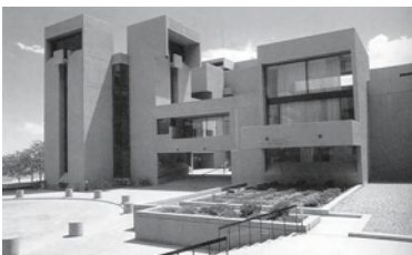
National Center for Atmospheric Research, Boulder, Colorado, USA; architect: I. M. Pei, 1961-67
