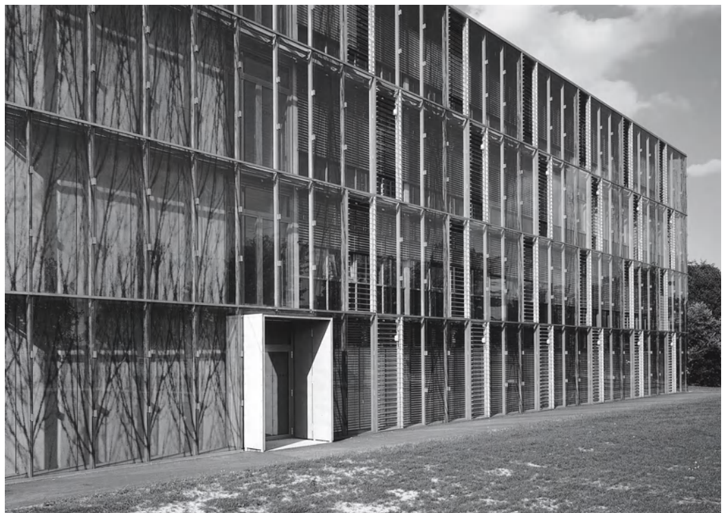
The glass façade provides the building with a coherent appearance | Accentuation of the cores by means of printed façade elements. Opened and closed louvers generate a vivid interplay
