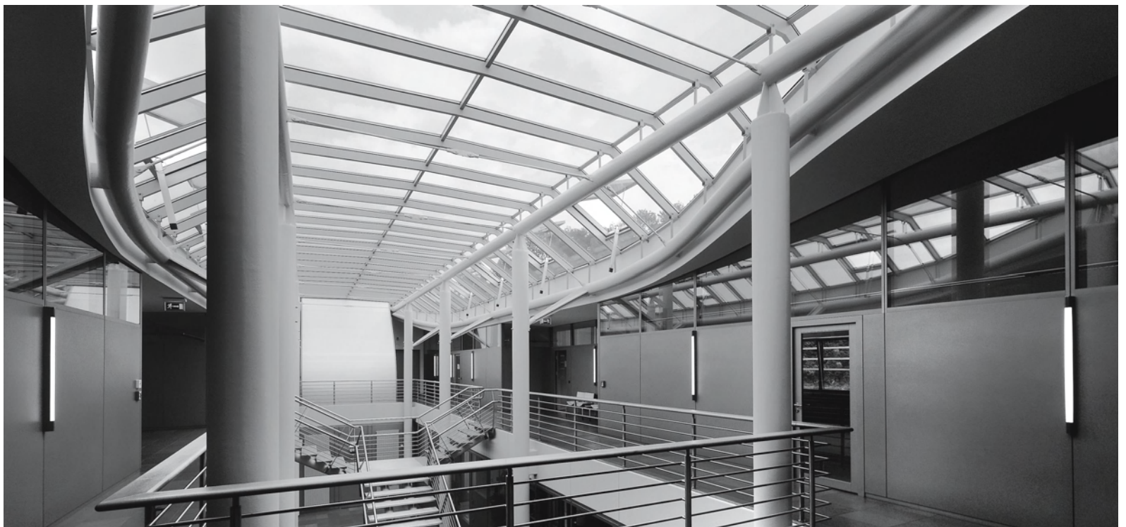
Atrium covered by skylights
