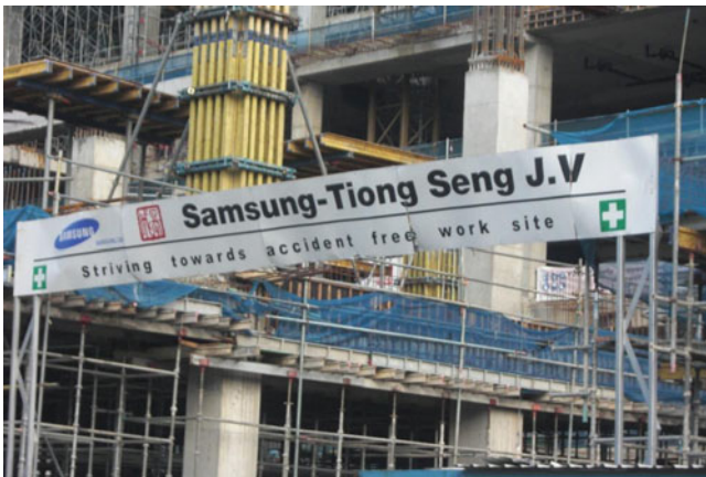
Fig. 3.2 A construction site near Farrer Park MRT Station with safety banner
