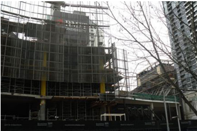
Fig. 3.1 Construction site in RMIT University, Melbourne ( author's photo )
