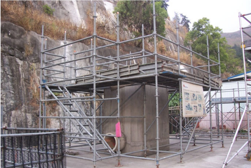
Fig. 6.8 Working at height training demonstration
