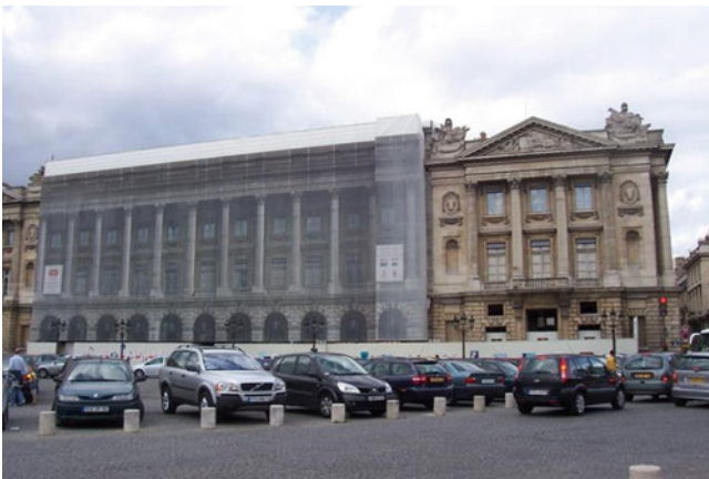
Fig. 3.3 A construction site in Paris with artistic picture covered ( author's photo )
