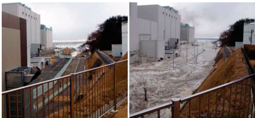
Fig. 7.44 Flooding of the Fukushima Daiichi NPS due to the tsunami
