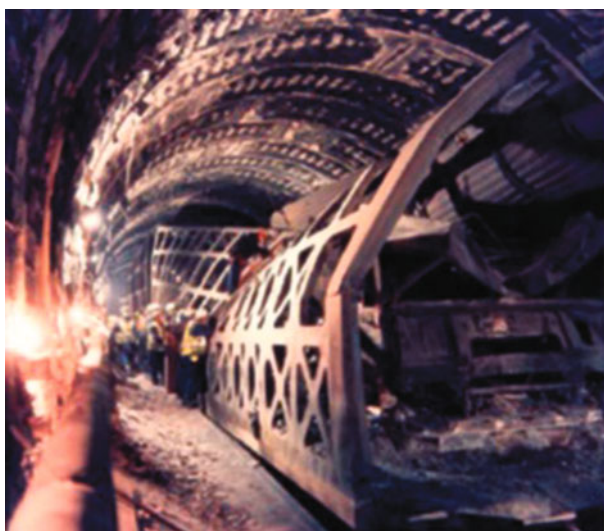
Fig. 1.11 Damage caused by the 1996 freight shuttle train fire in the Channel Tunnel (source http://www.tunneltalk.com )
