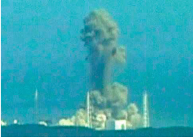
Fig. 7.45 Massive explosion of Unit 1
