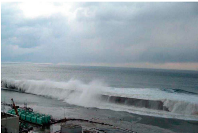
Fig. 7.43 The tsunami overtops the 10 m high seawall designed to protect the Fukushima Daiichi NPS
