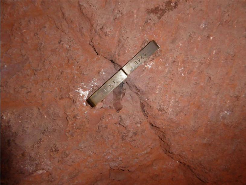
**PHOTO 14.6** A crack in the wall of Bet Raphael. The marker was placed across the crack in 1968 to monitor the rate of widening. Between then and 2014 it has widened by about 2 mm (2014)
