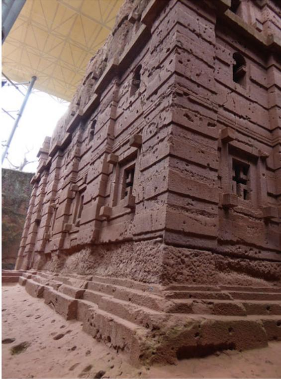
**PHOTO 14.7** Damage by water seepage to the base of Bet Emmanuel. The cover erected over the top of the church, of which a portion can be seen, has not addressed this problem. The Italians attempted to repair the damage with cement, which has now been removed (2014)
