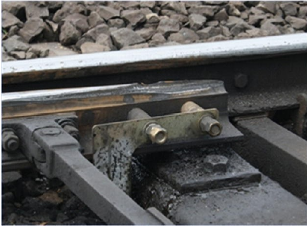
Figure 10.22 Damaged rail turnout and passage train.
