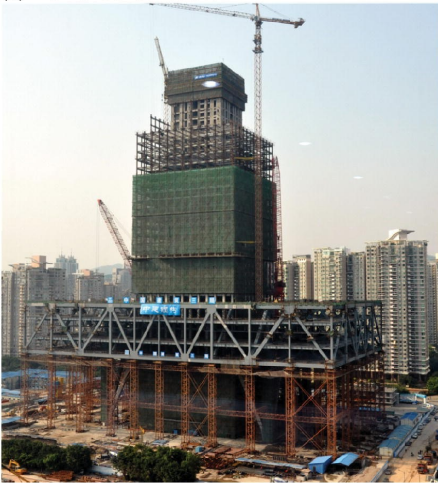
(a) View under construction
