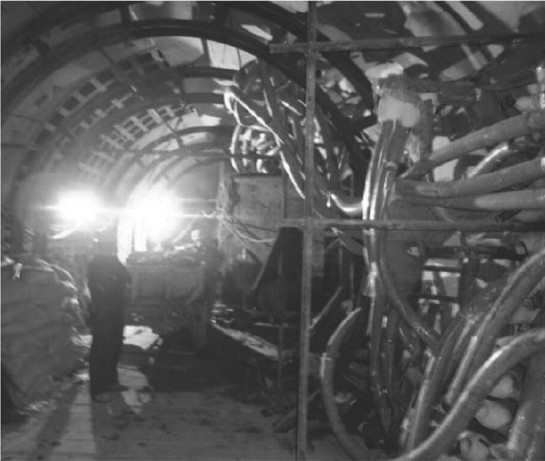
(a) Tunnel during construction
