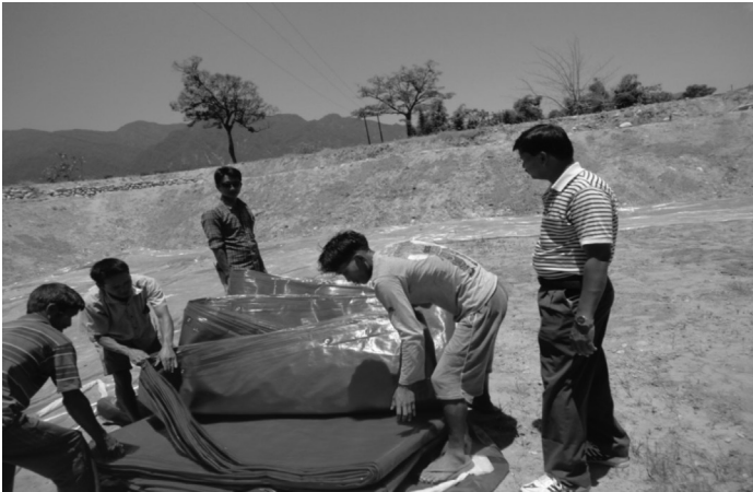
FIGURE 3.9 Unfolding of silpaulin film.
