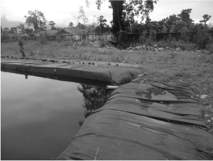
FIGURE 3.12 Pipe Spillway disposing of excess water.
