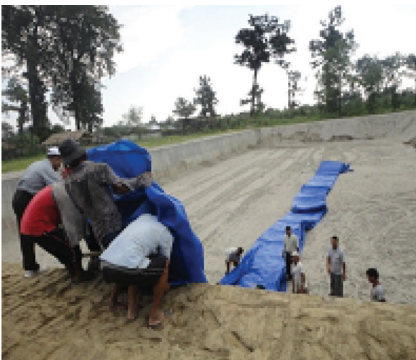
FIGURE 3.10 Spreading of silpaulin film.
