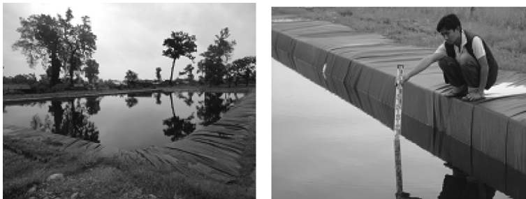
FIGURE 3.11 Harvested water in silpaulin lined pond.
