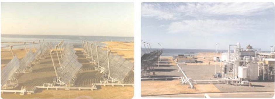
Figure 6: Pilot Solar Thermal Desalination Plant in Saudi Arabia
