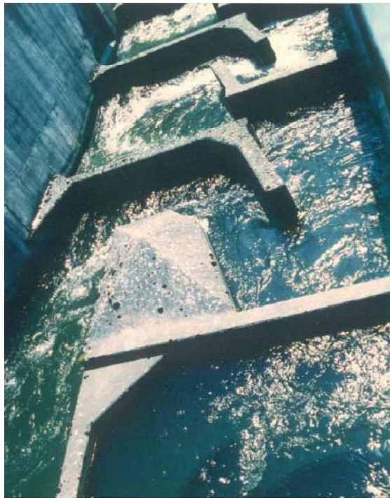
Figure 59. Fish ladder on the Bonneville Dam on the Columbia River. More than 1 million salmon swim through the fish ladder to pass the dam to upstream spawning grounds every year.
