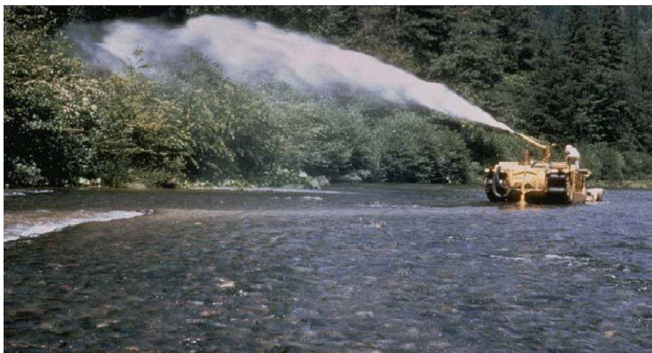
Figure 58. Hydroseeding of a streambank for restoration of understory riparian vegetation. Special tank trucks carrying seed, water, and fertilizer are used in the revegetation efforts (after FISRWG, 1997).
