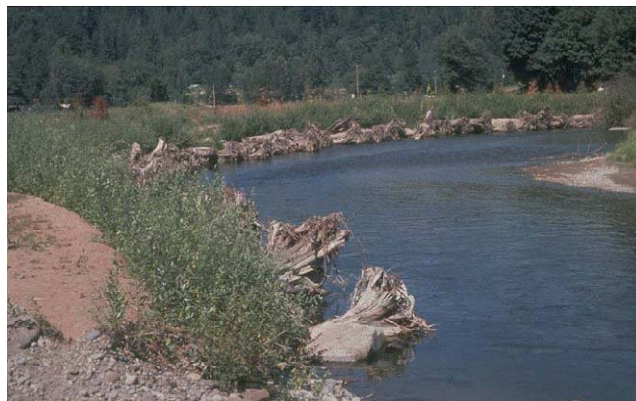
Figure 54. The protruding rootwads effectively reduce flow velocities at the toe (after FISRWG, 1997).
