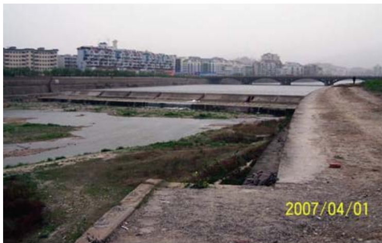
Figure 33. Riparian forest has been replaced by buildings and the banks are hardened with concrete in Guangyuan, Sichuan.
