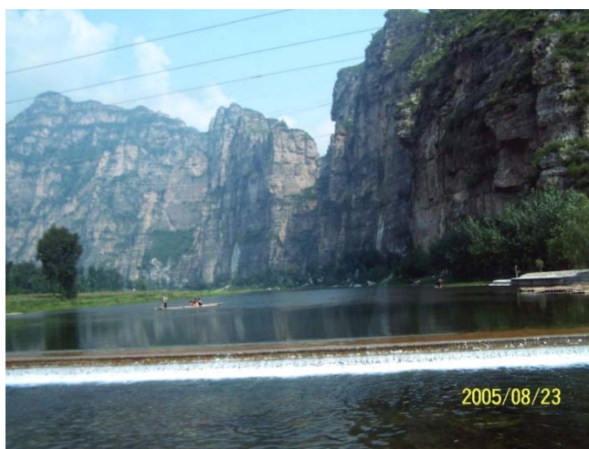
Figure 49. A weir placed on the Juma River in the suburbs of Beijing for creation and maintenance of a habitat with stable low current and high depth of water. In dry seasons the weir maintains a depth of water for fish and invertebrates to survive.
