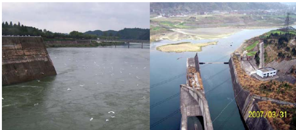
Figure 22. (a) Birds are searching for dead fish at the outlets of a hydro-power plant at which fish are killed when they swim through the turbine; (b) The Baozhusi dam on the Bailong River has cut off the flow and greatly affects the stream ecology in the lower reaches.
