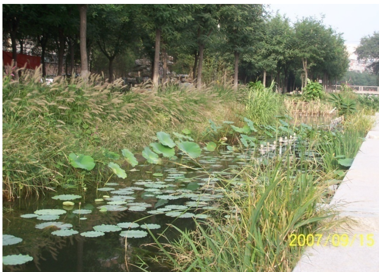
Figure 60. A layer of soil is placed on the hardened channel bed and banks on an urban stream in Beijing, and a vegetation bank and aquatic high plants have developed.
