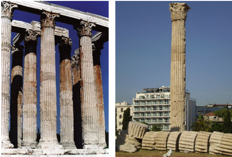
Fig. 24.1 Olympieion of Athens, Greece: Left: Columns and architraves at a corner; Right: A free-standing and a fallen column showing their multi-drum construction
