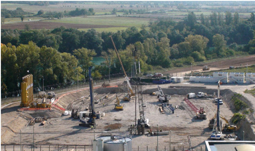
Fig. 14.9 Iceda (Le Bugey) site during construction
