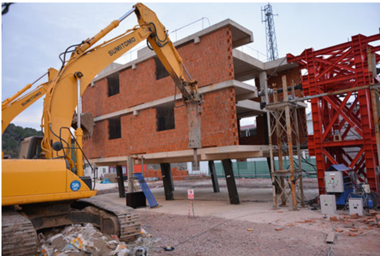
Fig. 22.11 Deformed shape of the FRP retrofitted building
