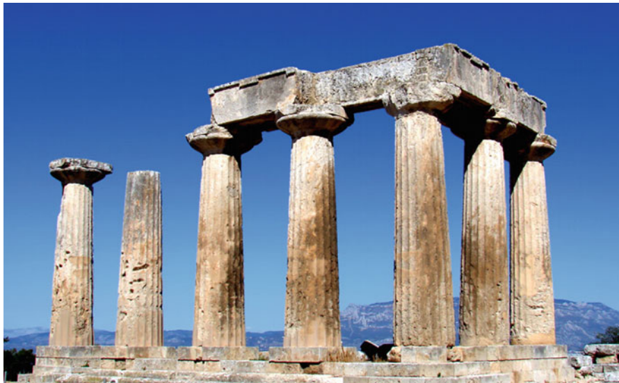
Fig. 12.2 View of the Temple of Apollo in Corinth, Greece. Its monolithic, free-standing columns support massive epistyles and the frieze atop, and the entire rocking frame remains standing for more than 2500 years in a region with high seismicity
