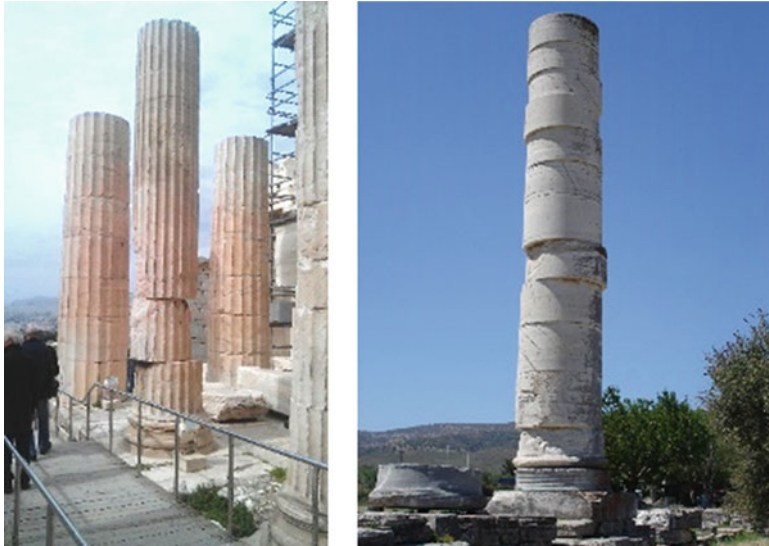
Fig. 24.9 Classical columns with significant drum dislocations. Left: Columns at Propylaea of the Acropolis of Athens, Greece; Right: Column of the temple of Hera in Samos, Greece
