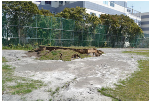
Fig. 16.11 Lateral spreading due to soil liquefaction and damage to pile foundations
