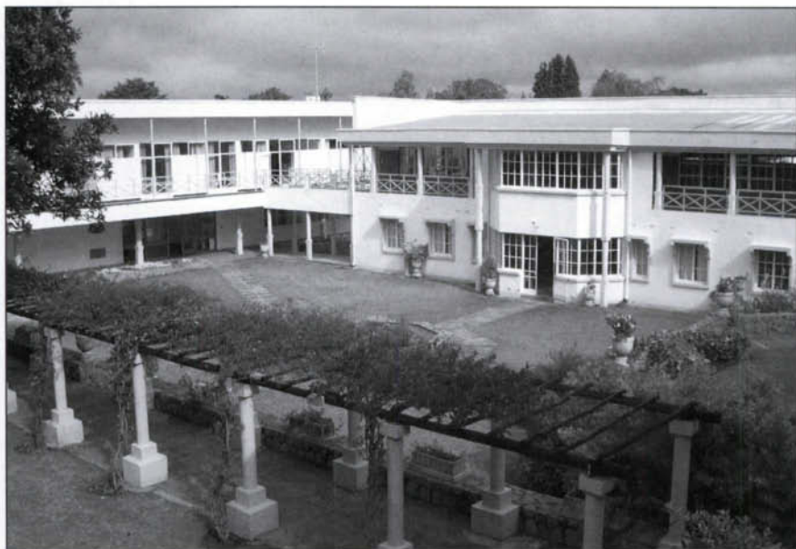
39. From above the entrance archway, into the new Humphrey Gibbs Court: the pergola in the foreground runs along the side of the chapel. The old 'admin block' (top left) still houses the masters' common room on the first floor; the new building on the right contains classrooms, computer rooms and offices. The old and new buildings are linked at first floor level; underneath is the walkway through to the Dame Molly Court.
