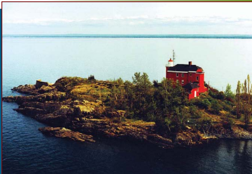
Marquette Harbor Lighthouse on Lake Superior, Marquette, Mich. Dale Fisher, U.S. Army Corps of Engineers
