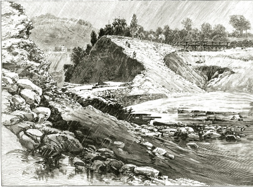
Fig. 7.3 The broken South Fork dam, as seen from inside the empty reservoir. The opening was about 130 m wide near the top; the spillway can be seen on the right just below the bridge. It took the flood surge roughly 53 min to reach Johnstown. Drawing by Schell and Hogan. (From Harper's Weekly , 1889.)
