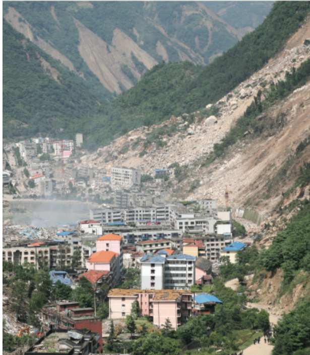
Figure 1.5 Rockslides triggered by the 2008 M7.9 Wenchuan, China, earthquake in Beichuan town (photo by Yueping Yin, China Geological Survey).
