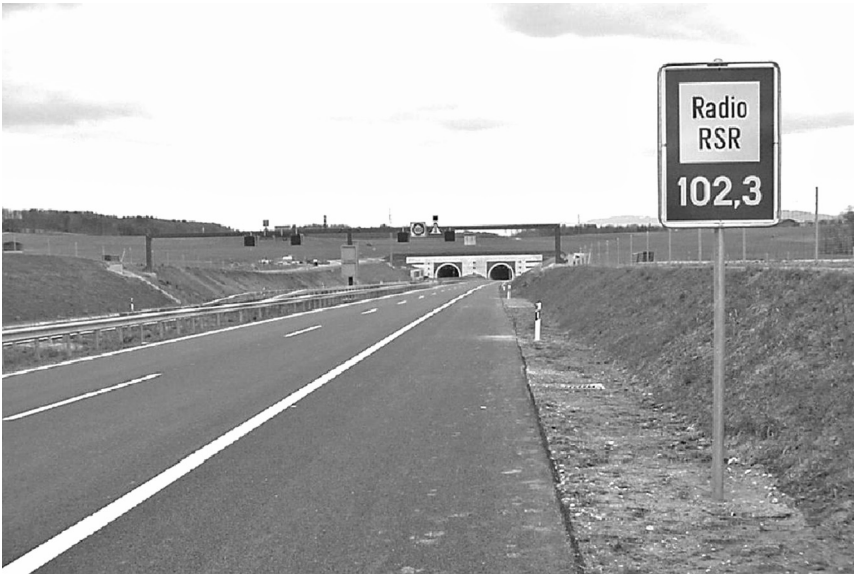
Figure 21.4 It is recommended that drivers in tunnels listen to the radio
