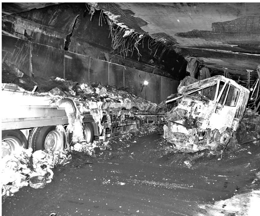
Figure 3.5 Photograph of the tunnel ceiling above HGVs 1 and 2
