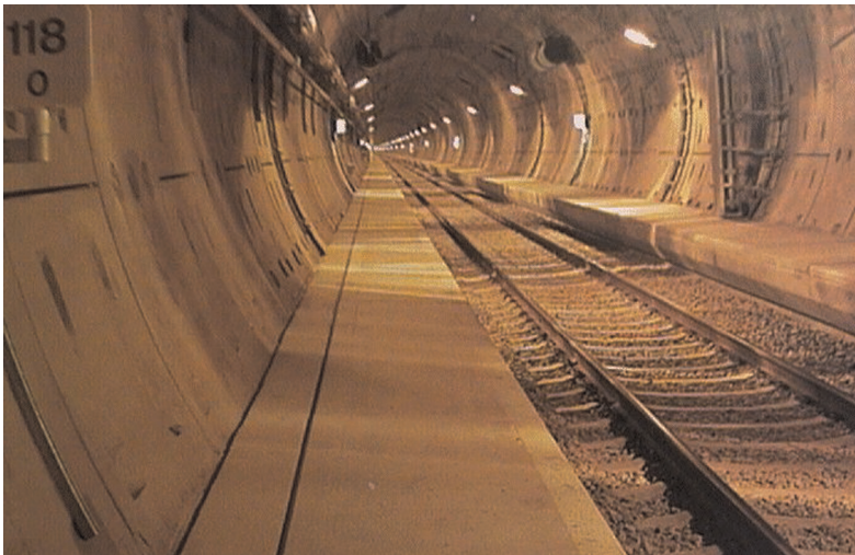
Figure 27.16 The Great Belt Tunnel
