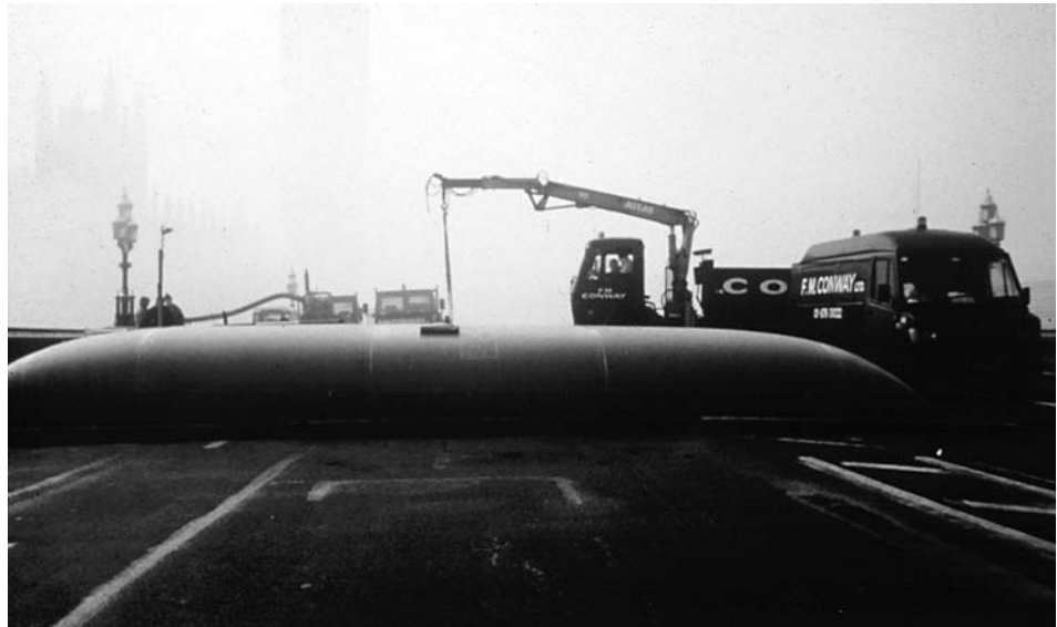
Figure 5.1 Pillow tank in use on Westminster Bridge, London.
