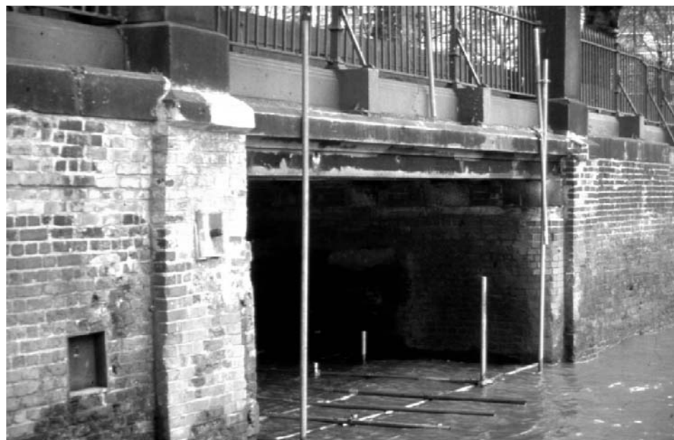
Figure D9 General elevation of the bridge
