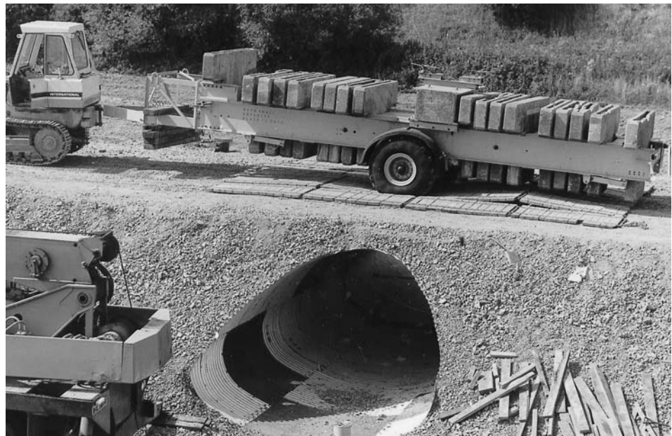
Figure 5.3 HB trailer used in loading test on a pipe arch culvert.
