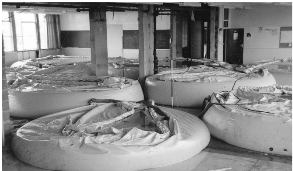
Figure 5.2 Flexible-dam-type water bag used to simulate floor loading.
