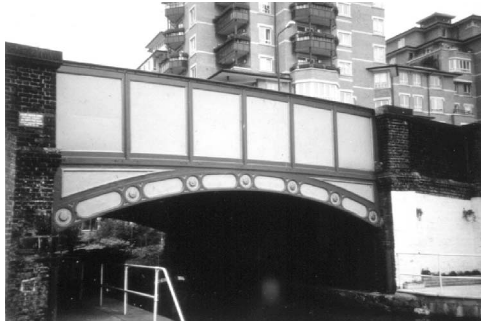
Figure D5 General elevation of the bridge.
