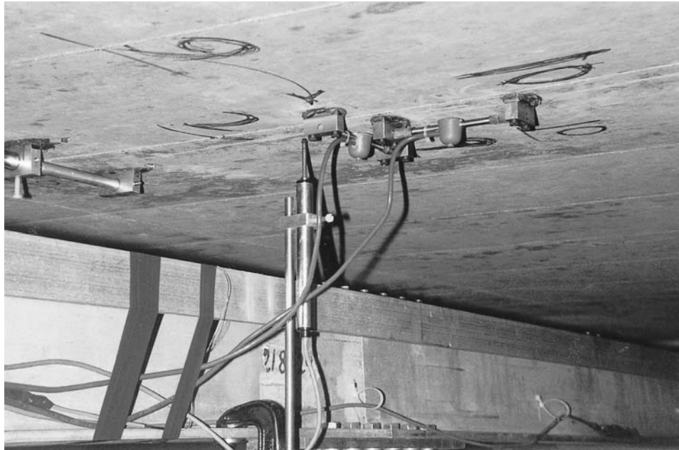
Figure 6.1 Bridge soffit showing vibrating strain gauges and LVDT displacement transducer.
