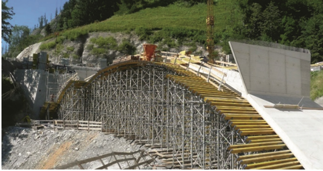
Fig. 1. Falsework of the arch of the Egg-Graben Bridge
