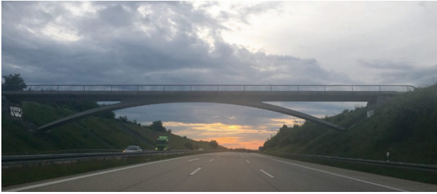
Fig. 1. Concrete arch overpass in Germany.
