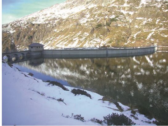
Fig. 20. The Lago Colombo dam at normal operating water level (November 8 th 2012). The spillway can be seen on left side
