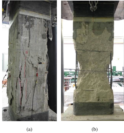
Fig. 7. Specimen damage at: the end of the test (a), after damaged concrete removal (b).
