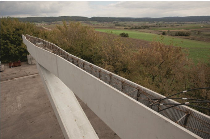
Fig. 16. Bridge girder with 70 mm prefabricated wall elements
