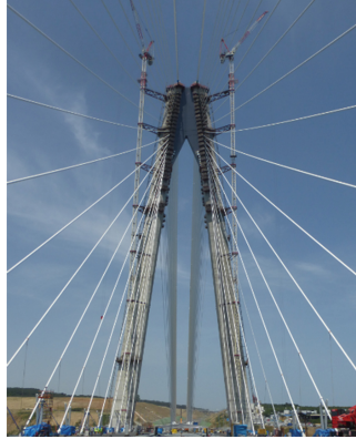
Fig. 20. 3 rd Bosphorus Bridge tower
