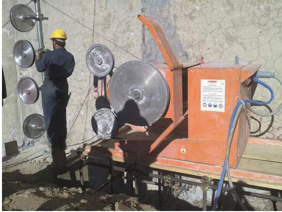
Fig. 11. The setup of cutting equipments and machines.
