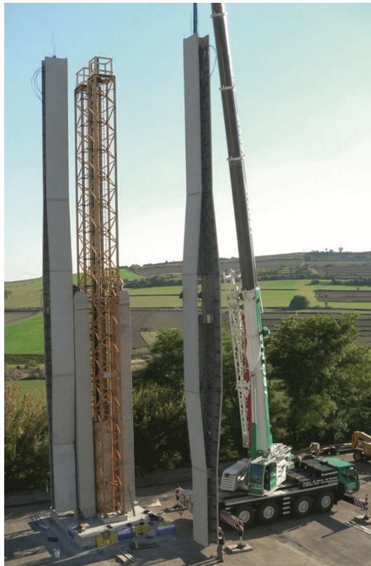
Fig. 12. The large-scale test structure during the mounting
