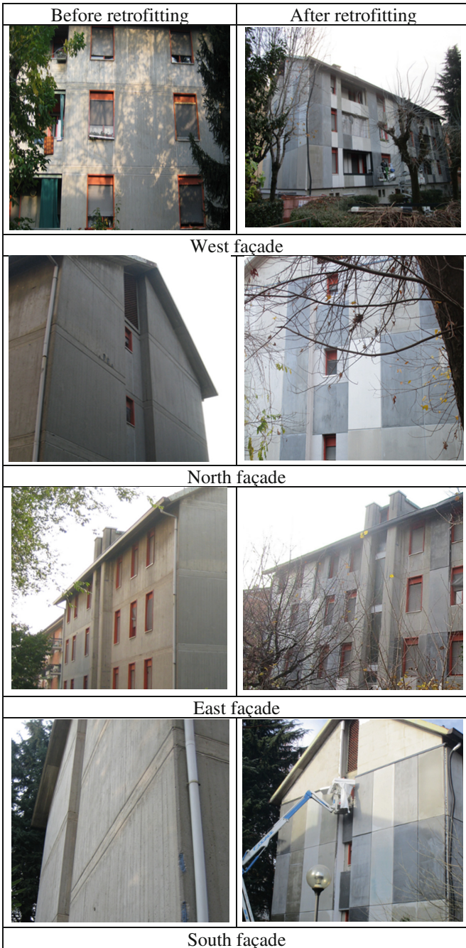
Fig. 7. Pictures before and after retrofitting
