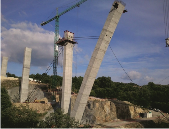
Fig. 4. Arnoia Bridge in Spain – lowering of arches (© VSL Hrvay Lifting, Switzerland)
