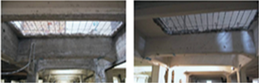
Fig. 1. Extracted beams T1 and T2 from existing RC buildings (1900s)
