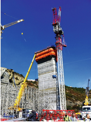
Fig. 19. The towers at the initial stage
