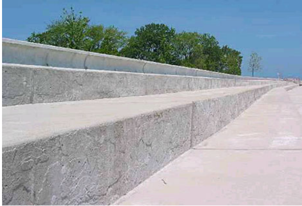
Fig. 4 A seawall protection to stop the Nile Delta being eroded by the sea
