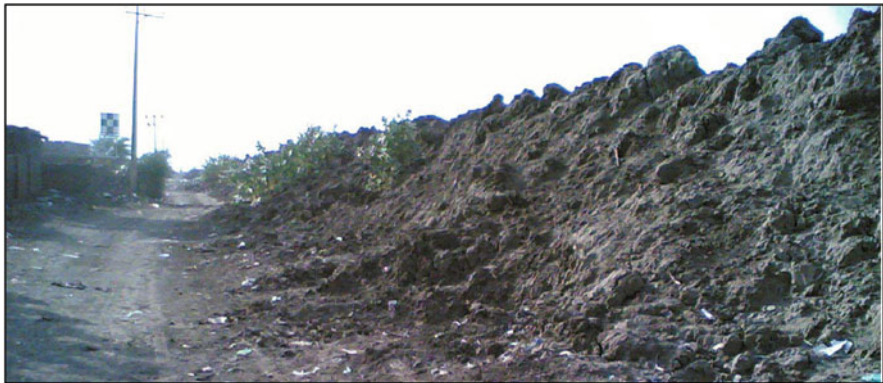
Fig. 4 Sediment excavated from the canal [8]
