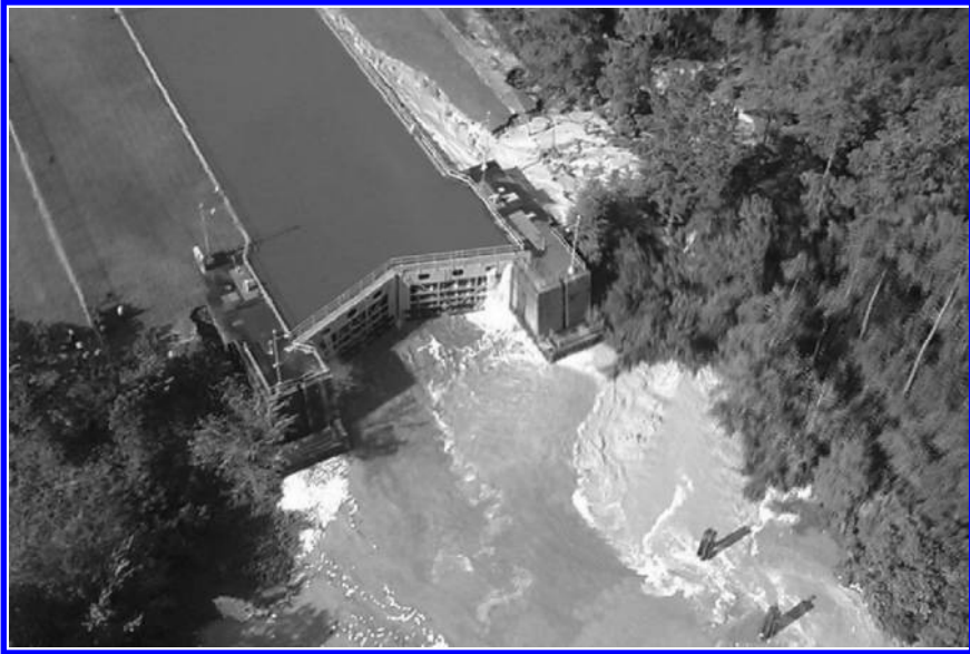
FIGURE 8.9 Pearl River lock and dam failure.
