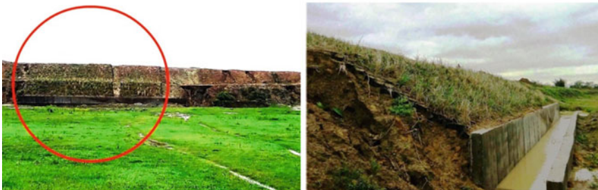
Fig. 11 20 m geocell protected stretch (circled) and a profile of the turfed slope
