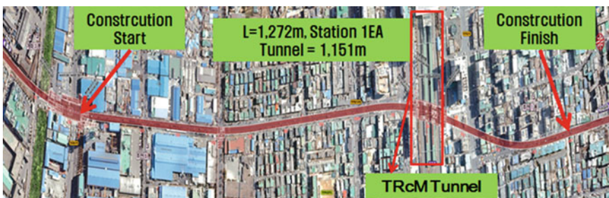
Fig. 10 View of Incheon Metro line No. 2, 218 station (L: 1.271 km)
