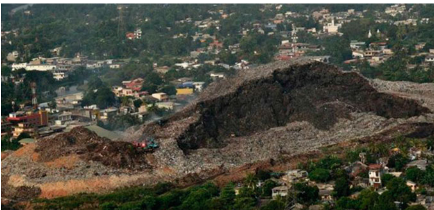
Fig. 1 Meethotamulla solid waste landfill: failed slope in the southwest direction (Source SLAF media)
