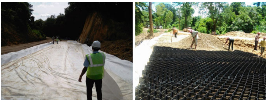
Fig. 7 Construction of pavement with geocells
