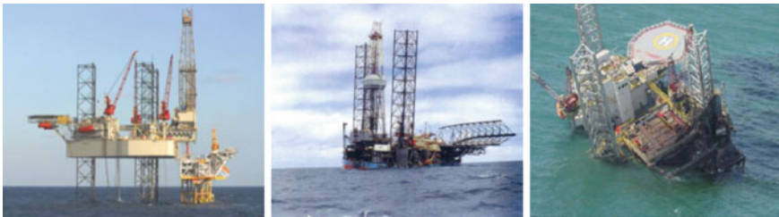
Fig. 2 Failure of jack-up units
