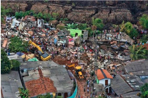
Fig. 2 Meethotamulla landfill slope failure in the southwest direction ( Source SLAF media)
