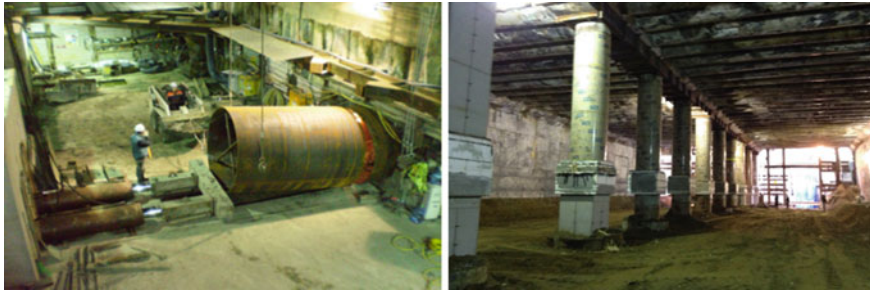
(a) Pressed-in steel pipe
