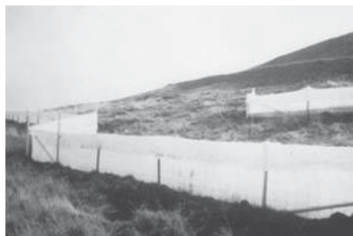
(a) Silt fences
