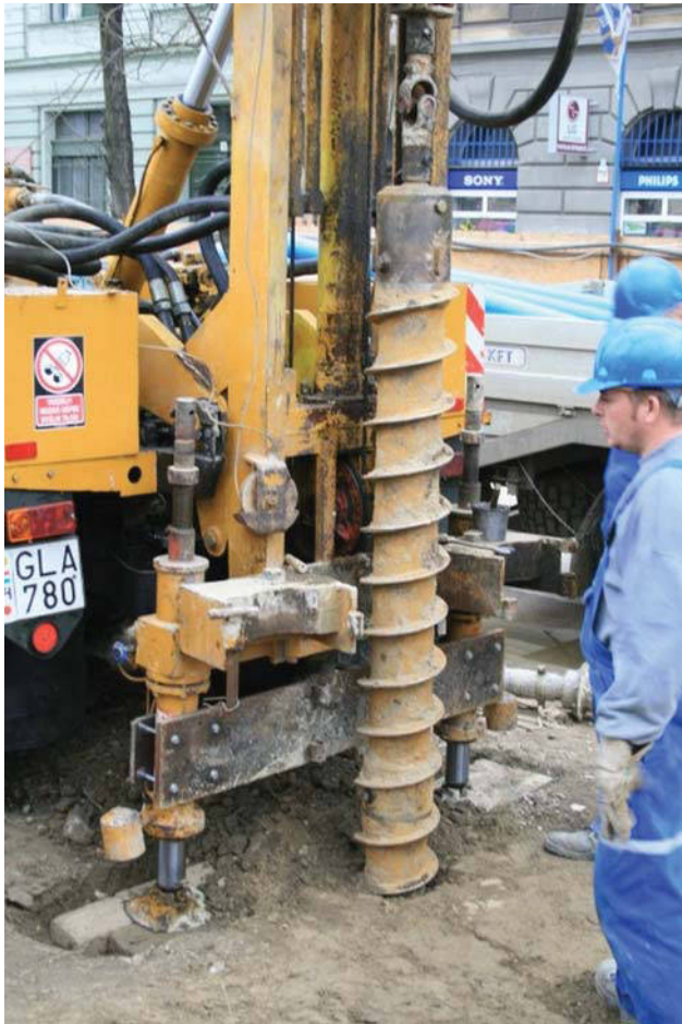
Figure 6.5 Hollow stem auger drilling method. (Courtesy of Geovil Ltd)
