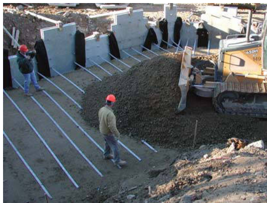
Figure 21.24 MSE wall. (Courtesy of The Reinforced Earth Company.)
