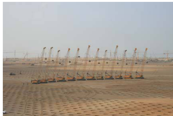
Figure 20.19 Dynamic compaction. (b: Courtesy of Menard Bachy Pty Ltd.)
