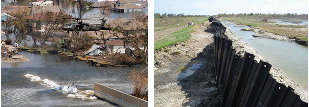
Figure 1.9 New Orleans levee failures during the Katrina hurricane in 2005. (Courtesy of United States Army Corps of Engineers.)
