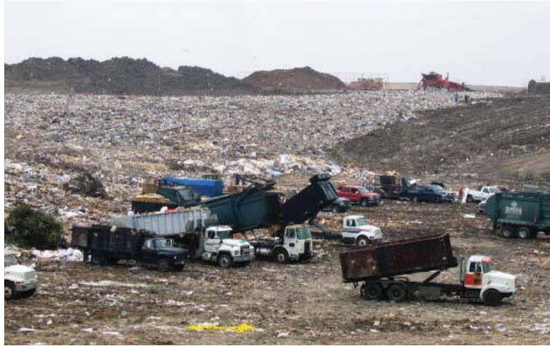
Figure 24.20 Landfill under operation. (Photo provided courtesy of the Texas Comptroller of Public Accounts from the Energy Report 2008, available at http://www.window.state.tx.us/specialrpt/energy/ )
