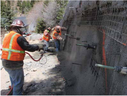
Figure 21.60 Soil nail wall construction (Courtesy of FHWA www.fhwa.dot.gov/publications/publicroads/11septoct/alongroad.cfm ).
