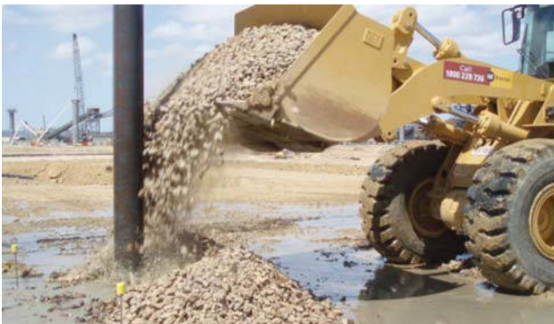
Figure 26.12 Stone column construction. (Courtesy of Menard Bachy, Inc.)
