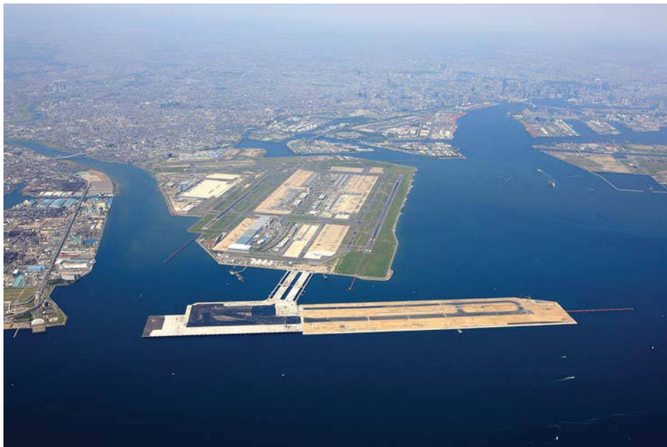
Figure 1.6 Extension of the Tokyo Haneda airport in 2010. (Courtesy of Kanto Regional Development Bureau, Ministry of Land, Infrastructure, Transport and Tourism, Japan.)
