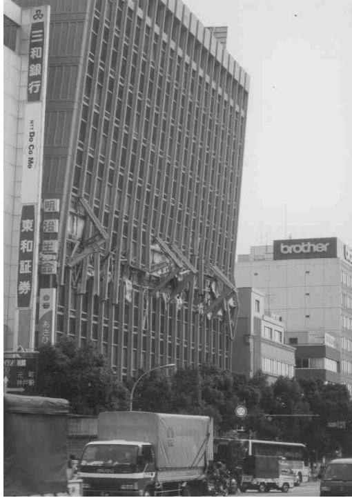
Figure 11.6 A building in Kobe, Japan that failed in the 1995 earthquake but did not collapse due to ductility in its beams and columns (© M. C. Griffith).
