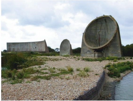
Fig. 4.1 Sound mirror—in Denge near Dungeness in Kent, Great Britain (in the area in front of the wall the researcher William Sansome Tucker installed 20 microphones for a better search for the direction of arrival of aircraft)
