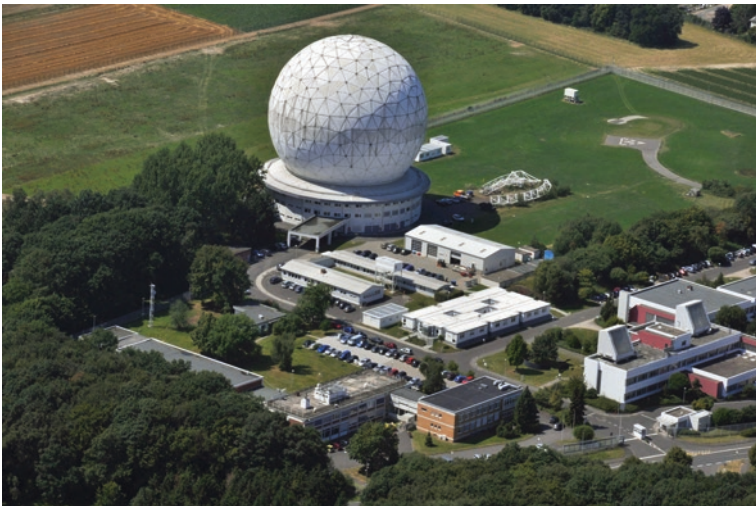
Fig. 9.24 The 47-m radome of the TIRA experimental radar characterizes the appearance of the Fraunhofer FHR site in Watchberg, near Bonn (Courtesy of Fraunhofer FHR)
