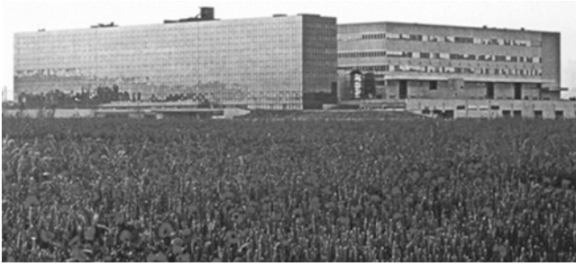
Fig. 7.45 The Contraves plant in Roma, Via Affile, 102
