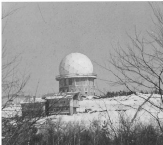
LONG RANGE RADAR INSTALLATION IN BULGARIA
