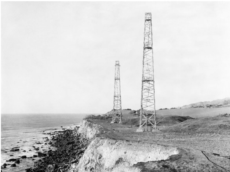
Fig. 4.10 Radar receiver towers and bunkers at Woody Bay near St Lawrence, Isle of Wight, England. This installation was a ‘remote reserve’ station to Ventnor CH
