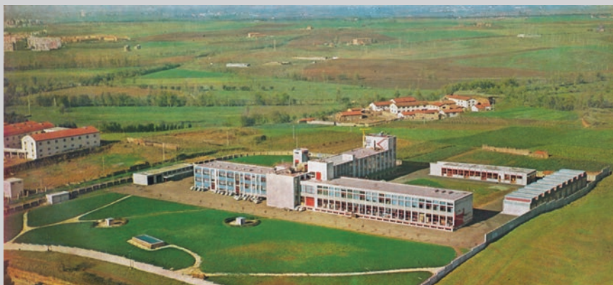
Fig. 7.31 The SINDEL plant (1959) in Via Tiburtina, Roma
