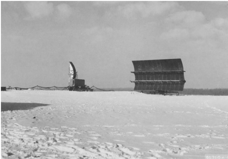
Fig. 5.16 The AN/CPS-1 microwave early warning (MEW) radar, deployed in time for D-Day on the south coast of England. On the left the British AMES Type 13 Mk III height seeking radar
