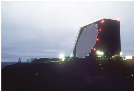
Fig. 9.11 The Cobra Dane installed in Alaska—the antenna has a diameter of 28.75 m and aims on the North Pacific area
