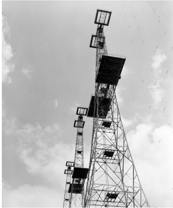
Fig. 4.8 AMES type 1 CH East Coast, 360 ft. transmitter aerial towers at Bawdsey CH station, Suffolk
