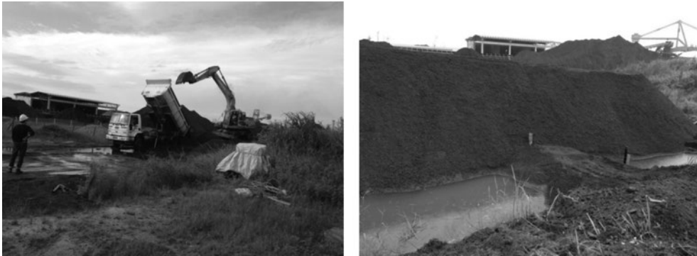
Figure 4.3 Typical moments of TKCSA test embankment construction (Hosseinpour, 2015)
