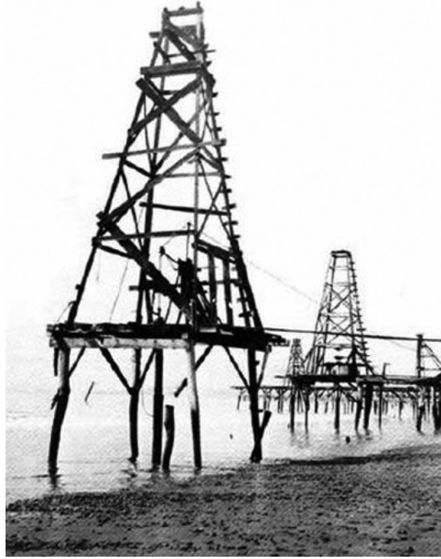
FIGURE 1.3 Production platforms in Summerland, California.
