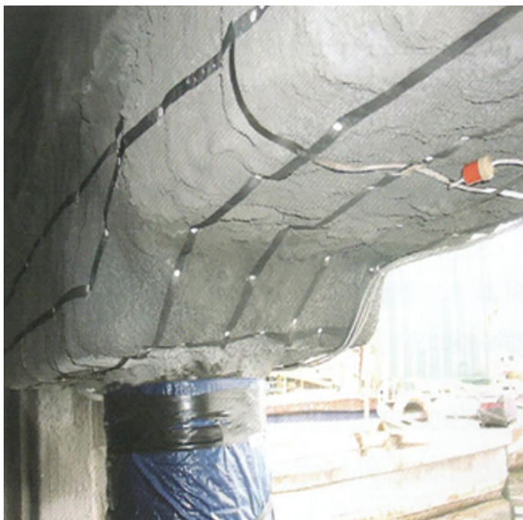
FIGURE 3.31 Cathodic protection to a rebar.
