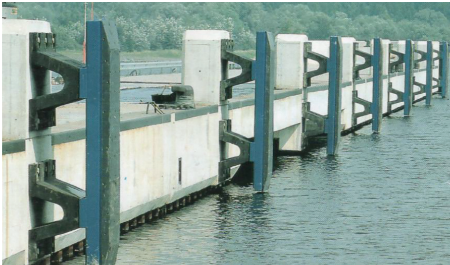
FIGURE 4.76 Arch fender.
