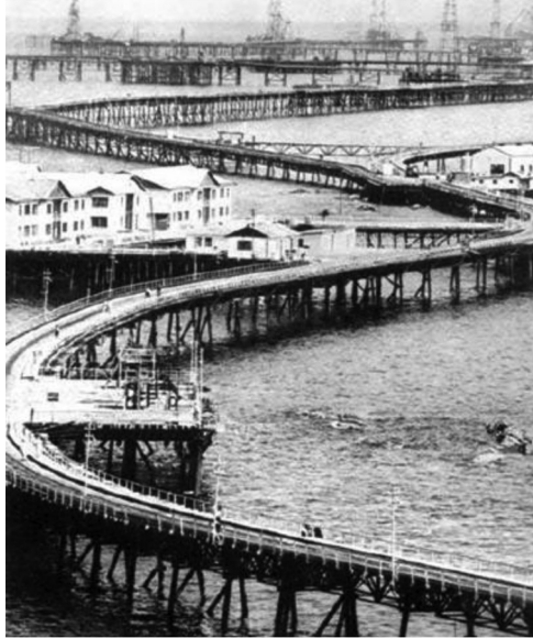
FIGURE 1.5 Drilling platforms in the Caspian Sea.
