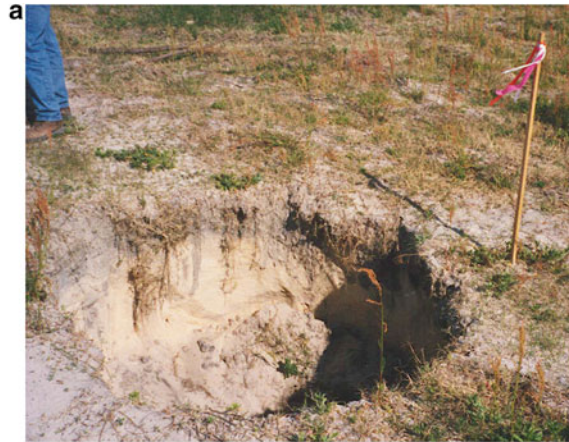
Typical small collapse feature associated with voids within the epikarst at a depth of about 12 meters
