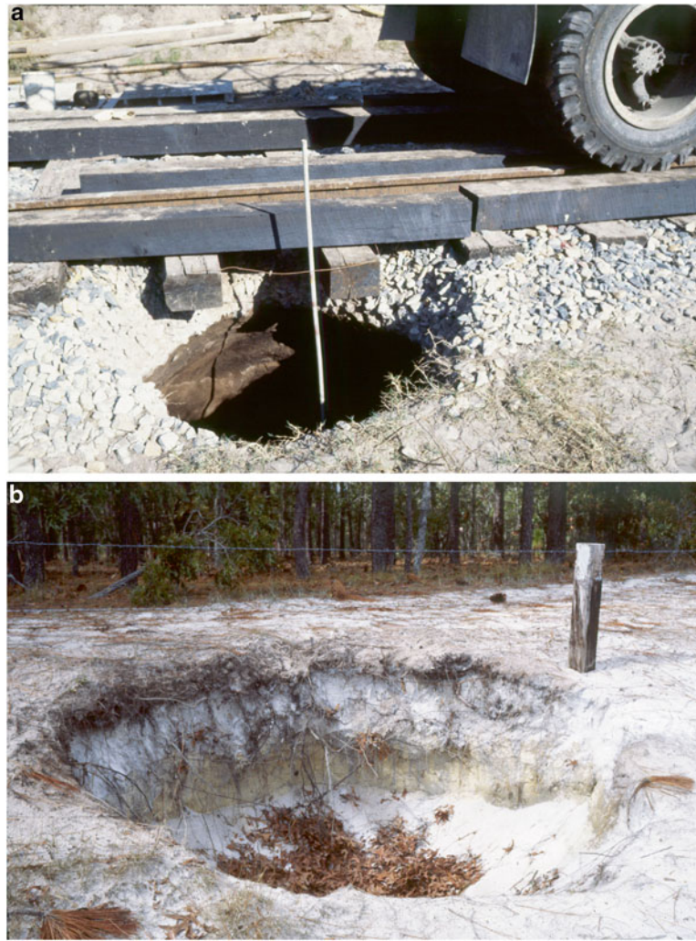
Fig. 8.3 Initial sinkholes at a site in North Carolina were quite small (<1 m in diameter) as a result of piping in sandy soils (a). Within a few weeks, these sinkholes would slowly enlarge to 3–6 m in diameter as the sandy soils continued to ravel (b)
