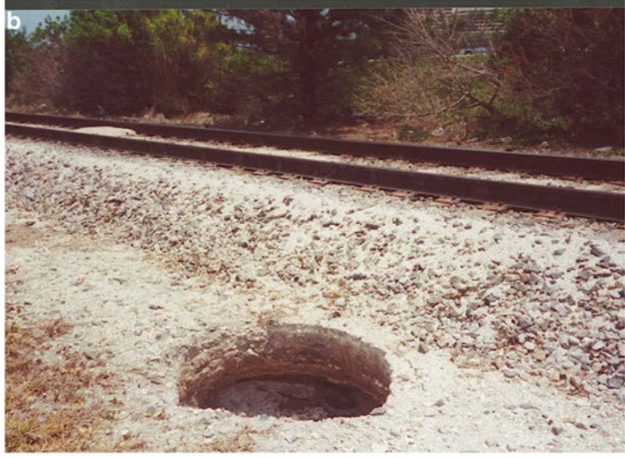
Fig. 3.5 Examples of small sinkholes are due to small pits or isolated cavities at or near the top of shallow rock (a) Sinkholes along roadway in Tennessee (b) Sinkhole along railroad in south Florida
