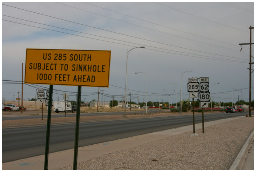
Fig. 7.12 Another site within the city of Carlsbad, New Mexico where salt was dissolved for drilling purposes has created a large cavity and a road sign alerts drivers to potential of sinkhole occurring in this area
