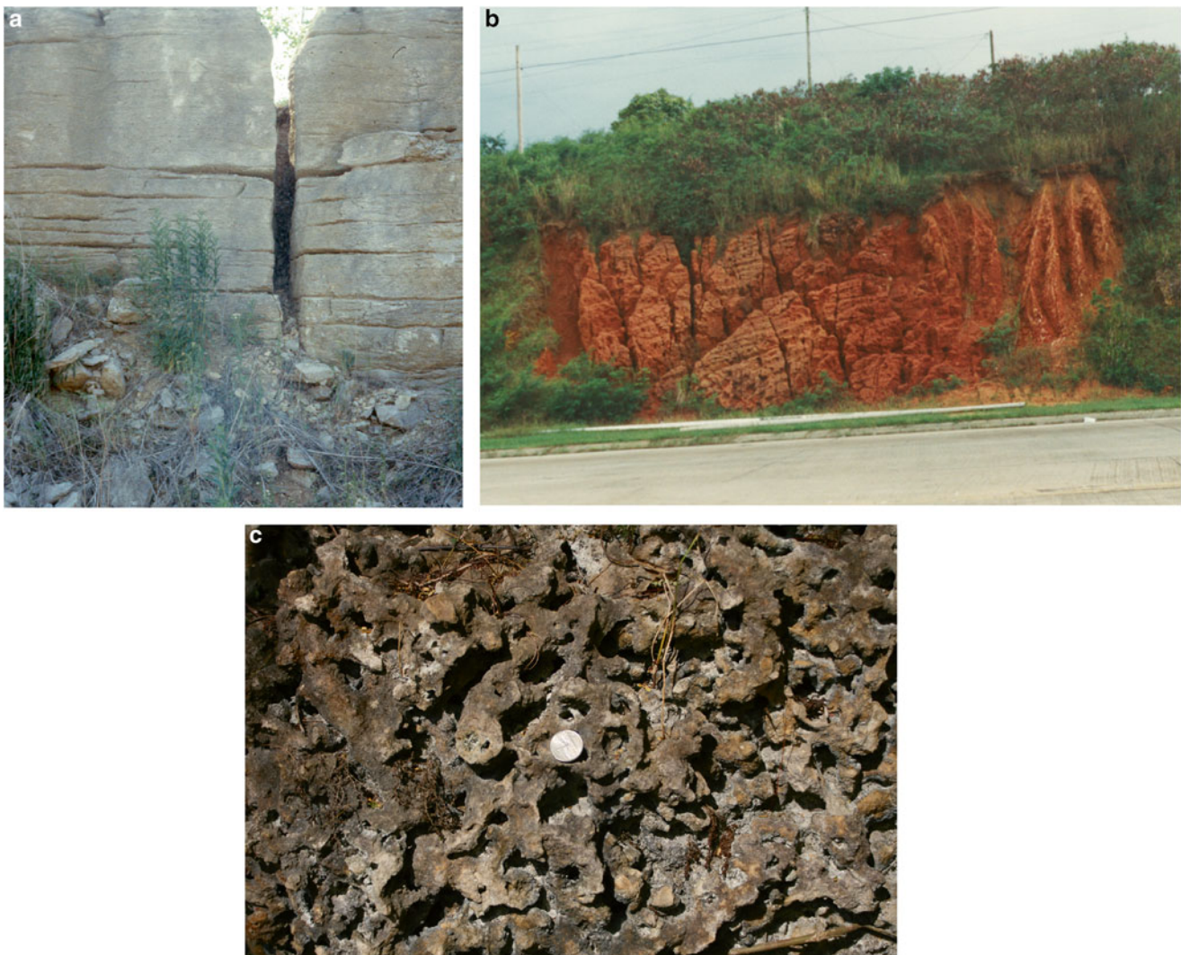
Fig. 2.5 Variations in limestone range from an older, massive strong limestone Kansas City, Kansas (a), a younger, highly weathered weak, almost friable limestone, in Puerto Rico (b) and a very young weaker, porous, Miami limestone (c) in south Florida
