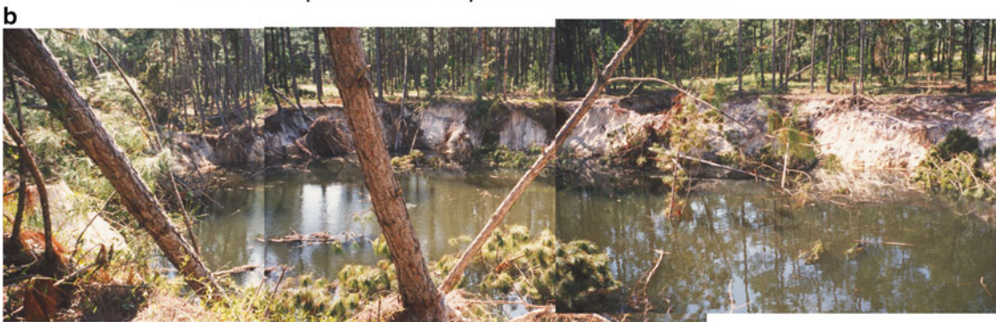
One of the large collapse features associated with caverns within the limestone at depths of about 30 to 60 meters below grade
