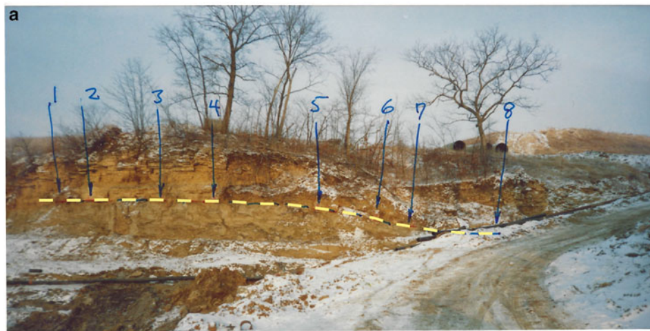
Note dipping layer exposed during excavation
