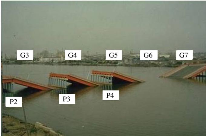
Fig. 1.3 Photo of the Showa bridge after the 1964 Niigata earthquake (Hamada 1992)
