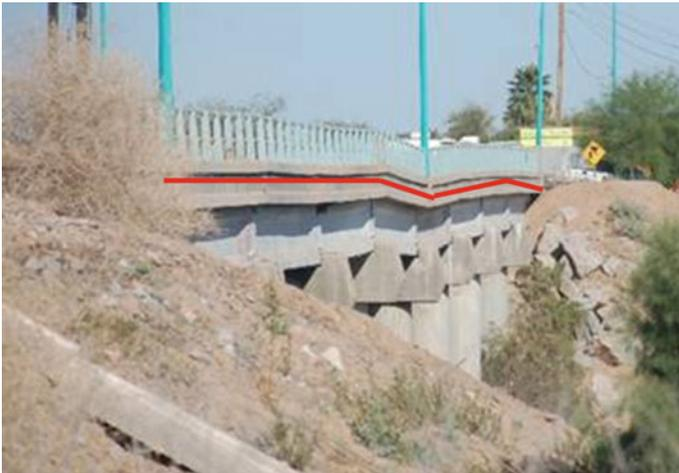
**Fig. 1.8** Downdrag induced settlement of road bridge piles in the 2010 Baja California earthquake (Stewart and Brandenberg 2010)
