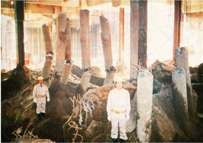
Fig. 1.5 The pile foundation of the NHK building after excavation (Hamada 1992)
