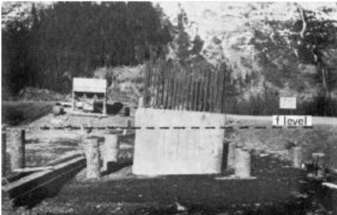
**Fig. 1.2** Failure of the pile foundation of 605A bridge (Ross et al. 1973)
