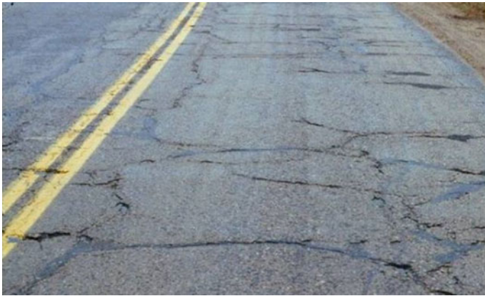
Fig. 1.16 Photograph of surface aging. (Source Road Science, a Division of ArrMaz)
