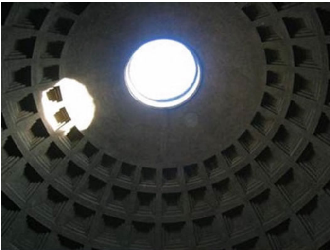
Fig. 1.5 The Oculus in the Dome of the Pantheon (note the inlaid pattern in the concrete ceiling)
