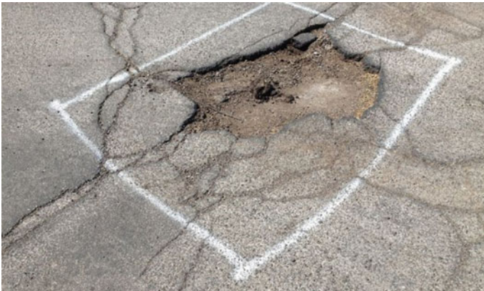
Fig. 1.24 Photograph of potholing. ( Source Road Science, a Division of ArrMaz)
