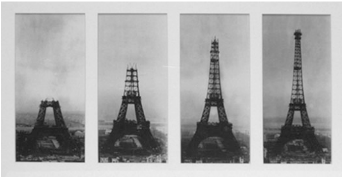
Fig. 1.12 Photographs of the Eiffel during construction
