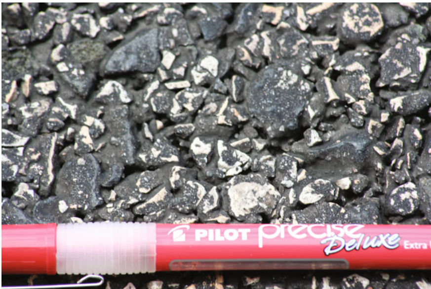
Fig. 3.12 A PFC mix on the pavement surface with exposed aggregate surface a few weeks after it was opened to traffic (Photograph by A Bhasin)
