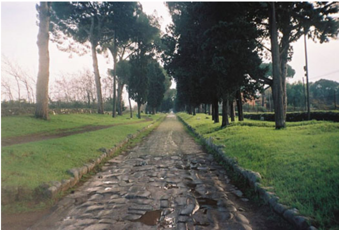
Fig. 1.3 Via Appia today (note the crowning of the roadway)
