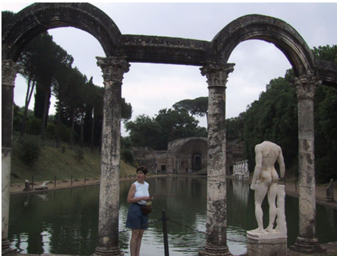
Fig. 1.7 Beams and Arches connecting columns adjacent to the Canopus at Hadrian's Villa
