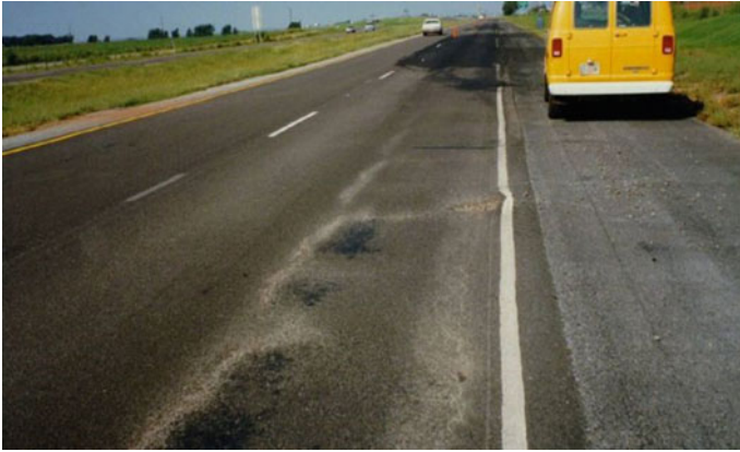
Fig. 1.23 Photograph of stripping. ( Source Road Science, a Division of ArrMaz)
