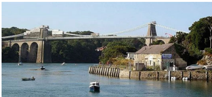
Fig. 1.10 Photograph of the Menai Suspension Bridge
