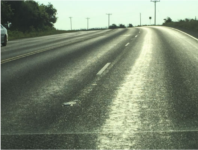
Fig. 8.11 Typical example of a pavement section with bleeding (Photograph taken by A Bhasin)
