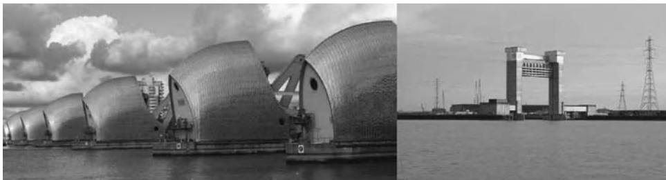
Fig. 23.2 The Thames Barrier (left) and Barking Barrier (right).
