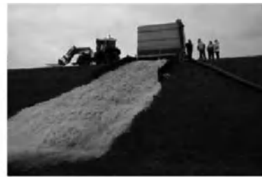
Surface erosion due to overtopping (floodsite)
