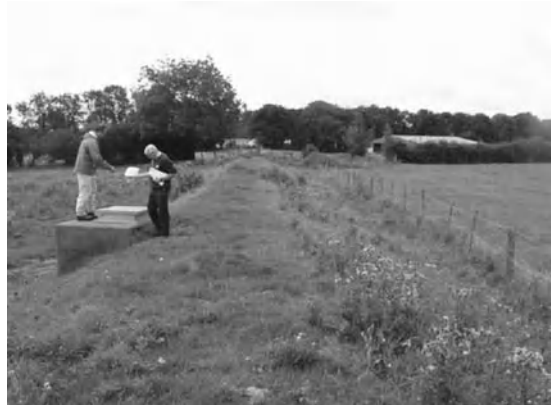
Fig. 6.8 Embankment length and view along crest.
