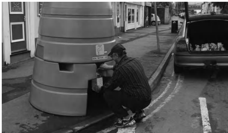
Fig. 21.3 Bowser supply in Gloucester, following flooding of Mythe water treatment works. Photo: L. Fewtrell.
