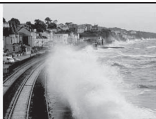
Hazards to railway
