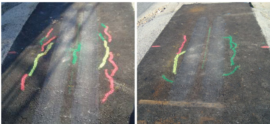
Fig. 1.18 Final condition of structure P1 without grid (left) and structure P3 with Tri-Ax grid (right) [39]
