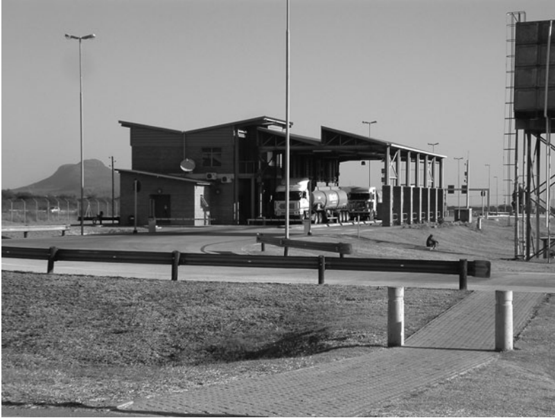
Figure 16.3 Covered static scale and TCC building, Zebediela, South Africa (Source: SANRAL)
