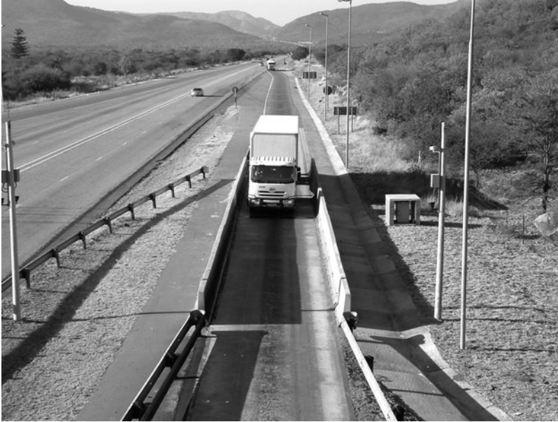
Figure 16.2 Typical screener lane installation, Zebediela, South Africa (Source: SANRAL)
