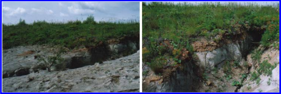
Figure 7.10 Grey flotation tailings covered by a thin soil layer: extensive water erosion.
